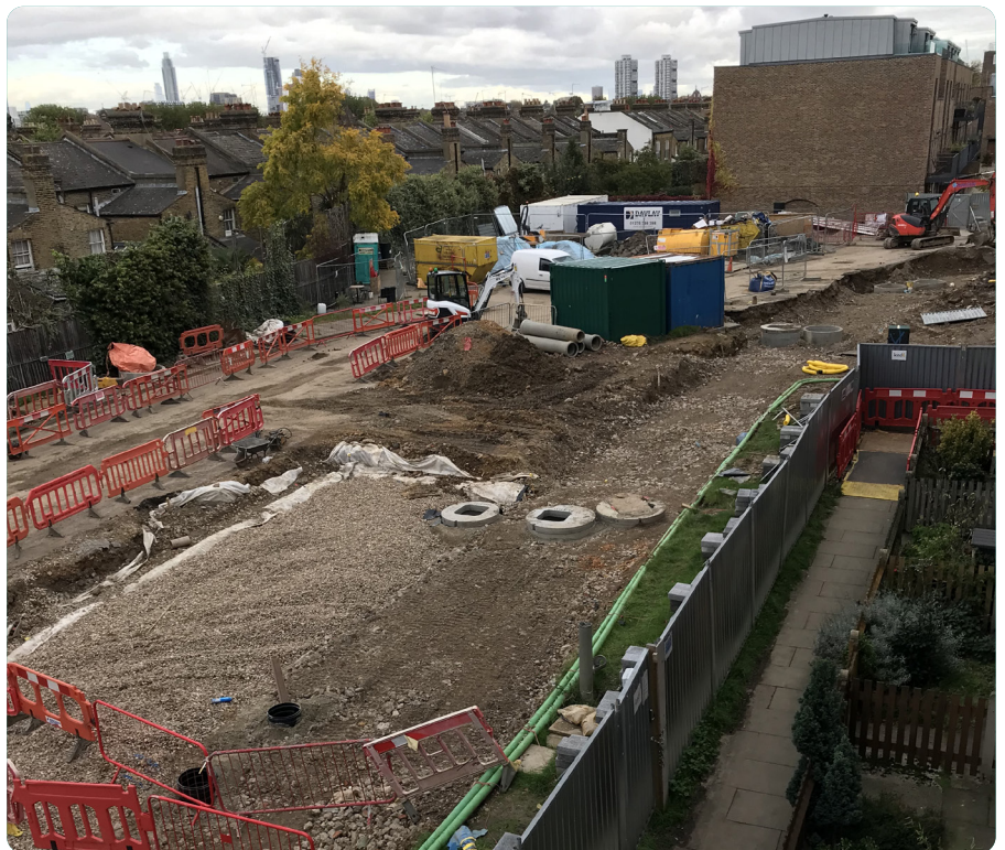
Backfilling to road level
