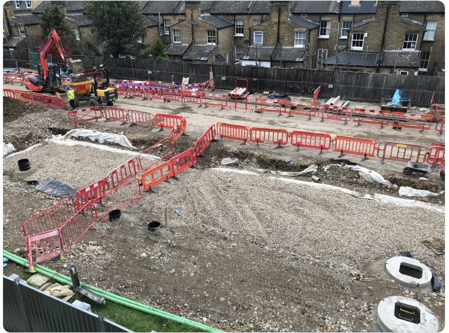
Backfilling to road level
