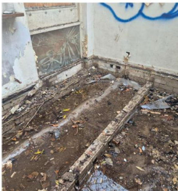
Figure 9: Photograph of the concrete slab below the ground floor joist structure
