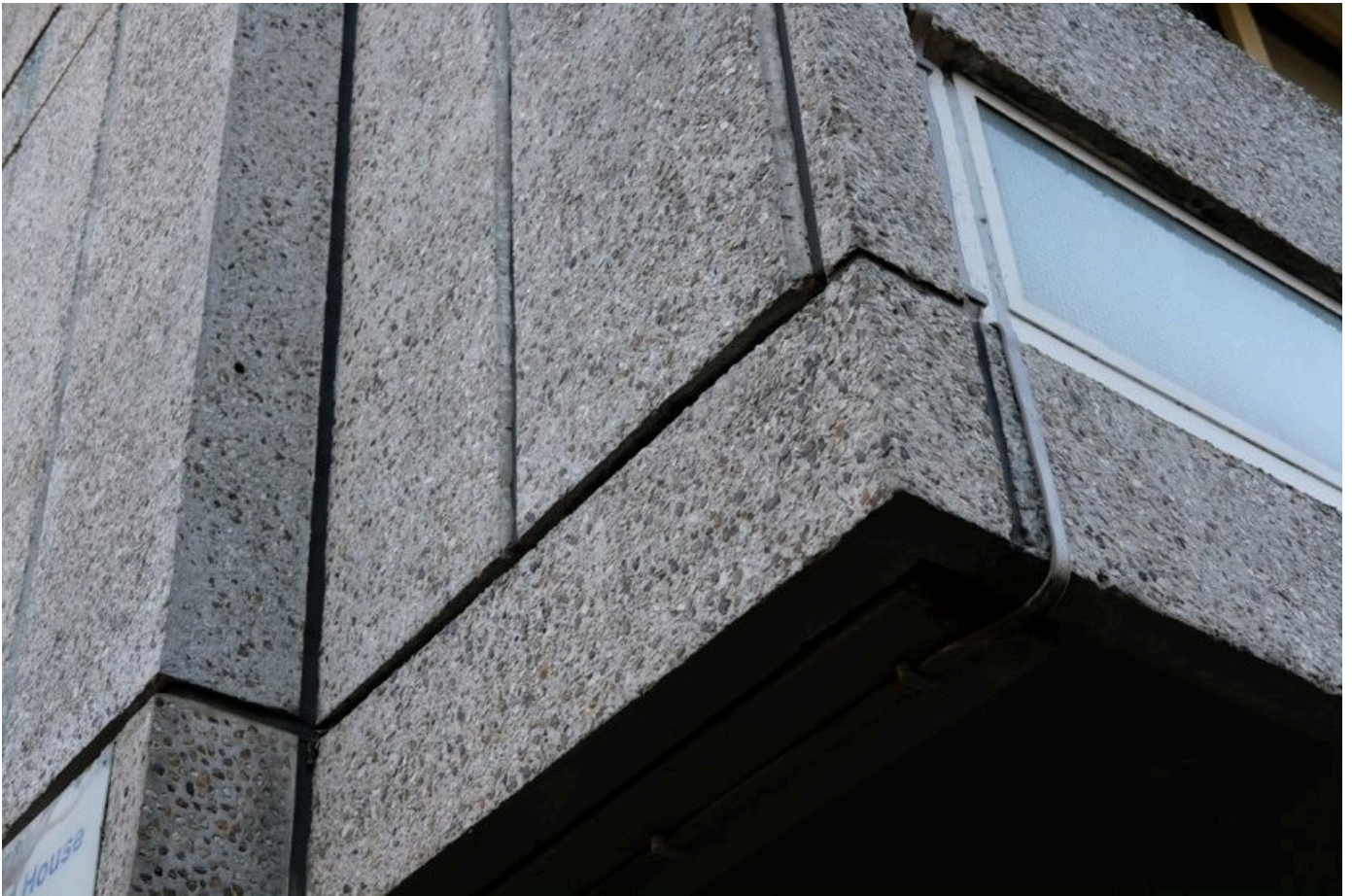
Fig. 91: Detail showing the Dorset shingle and Derbyshire spar exposed aggregate
