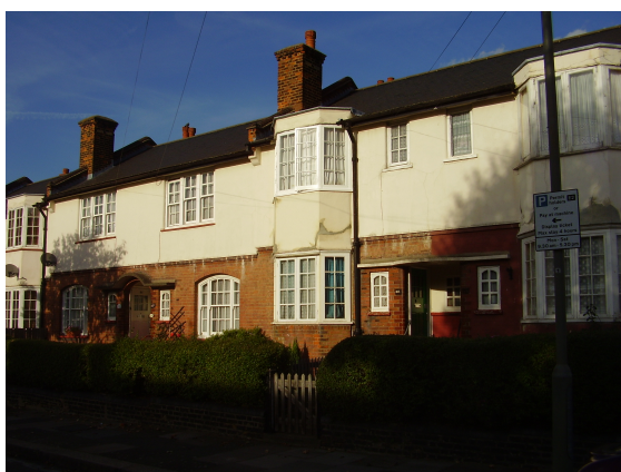
Picture 1.5 Terrace of cottages constructed of yellow stock brick with roughcast render on the upper storey
