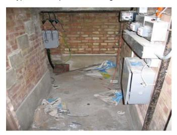
The intake cupboards are dusty and there is evidence of litter on the floor, providing good bedding material for rats. There may also be items stored in the room which prevent access to meters and other equipment.
