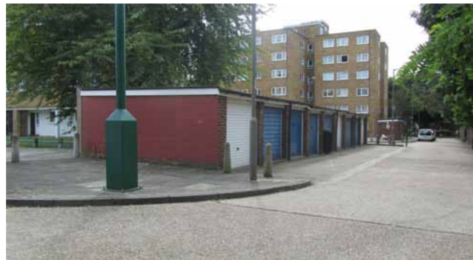
5 - View towards entrance from Aldrington Road
