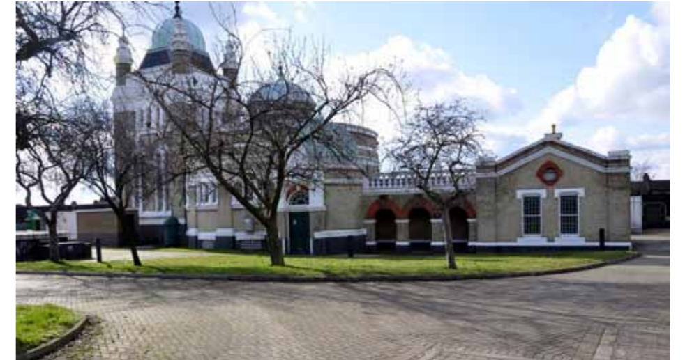
3. Streatham Pumping Station
