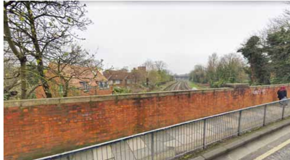
2. View of the railway tracks from Mitcham Lane
