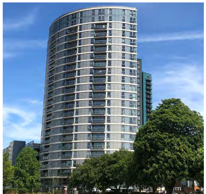
Fig. 298: Mature planting and large open spaces help to integrate and can better accommodate tall buildings
