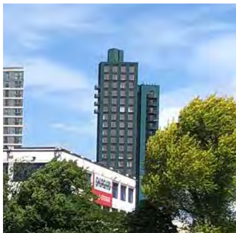
Fig. 353: 11 Mapleton Crescent scheme from King George's Park
