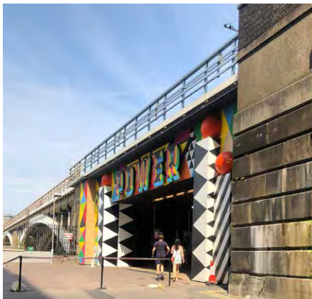
Fig. 95: Colour and vibrancy created by artistic Grosvenor Arch gateway under Battersea Bridge
