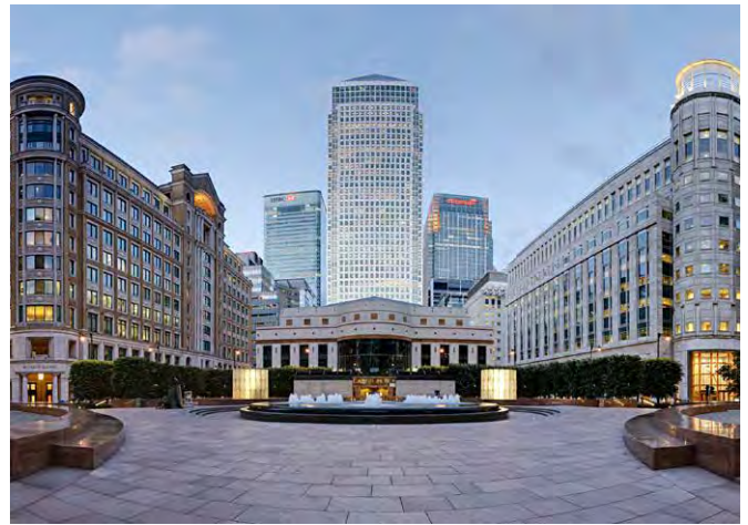
Fig.294: One Canada Square, Canary Wharf was designed as a landmark with views framed by surrounding background buildings © Photo by DAVID ILIFF. License: CC BY-SA 3.0
