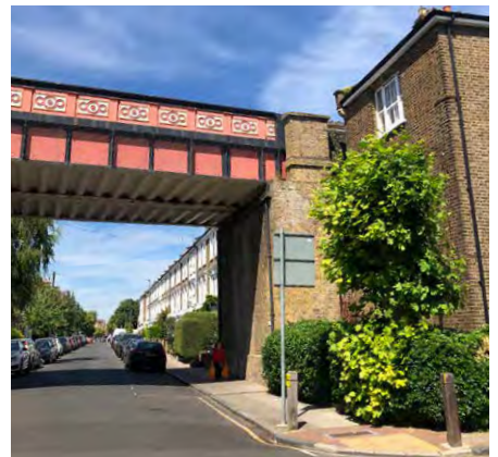
Fig. 161: Railway bridge at Fawe Park Road
