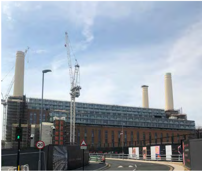
Fig. 93: The iconic Battersea Power Station during redevelopment
