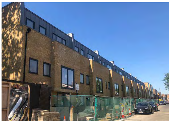
Fig.318: Precedent new build terrace row along Balham New Road
