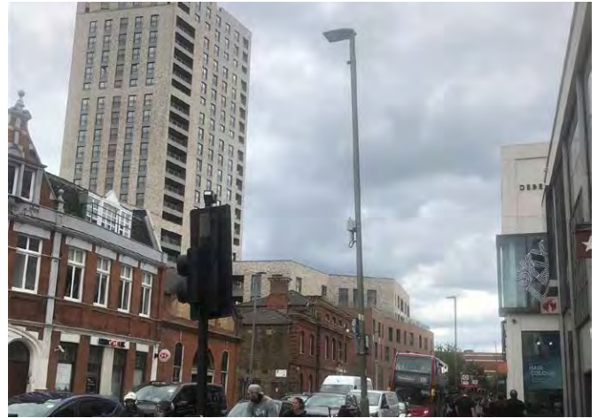
Fig. 297: This mass and height of this building adversely dominates the consistent street scene along Wandsworth High Street
