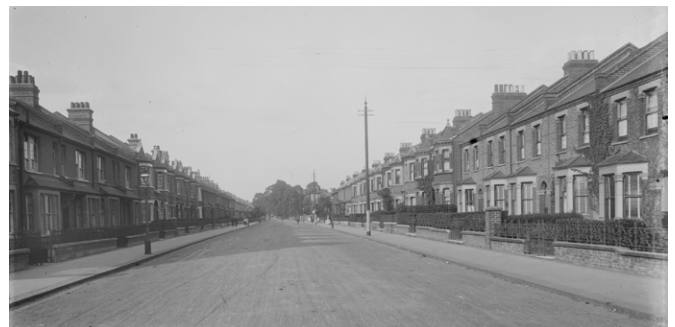
Fig. 37: Burntwood Lane in Earlsfield, 1915 © Wandsworth Heritage Service
