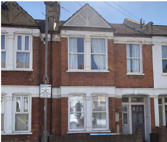
Fig. 197: Two storey period terraces on Totterdown Street
