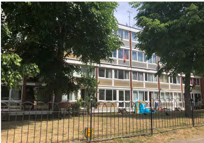
Fig. 381: Mid-rise estate block in Alton East, Roehampton
