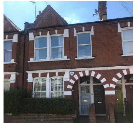
Fig. 213: Typical period terraces on Welham Road, with intact front boundary walls and hedges
