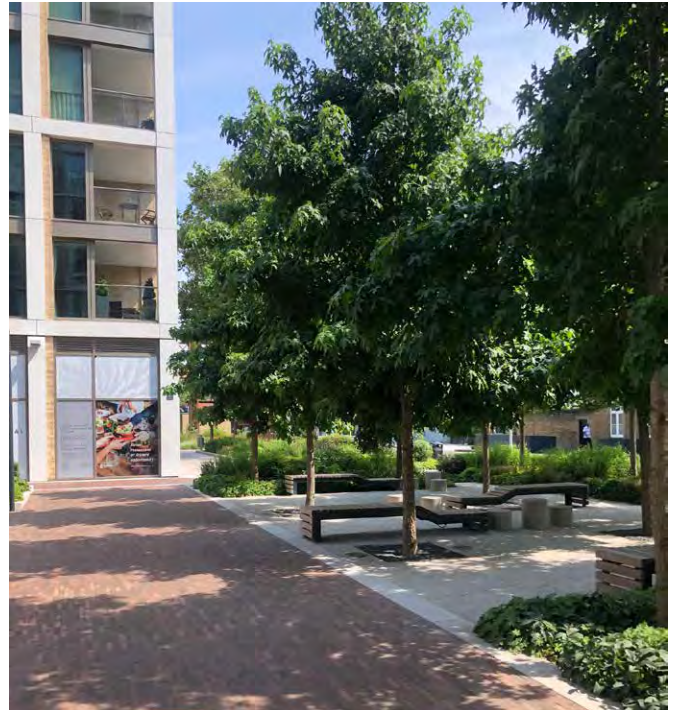
Fig.310: Attractive public realm with quality materials, integrated seating and a generous allocation of space at a new residential development at Prince of Wales Drive
