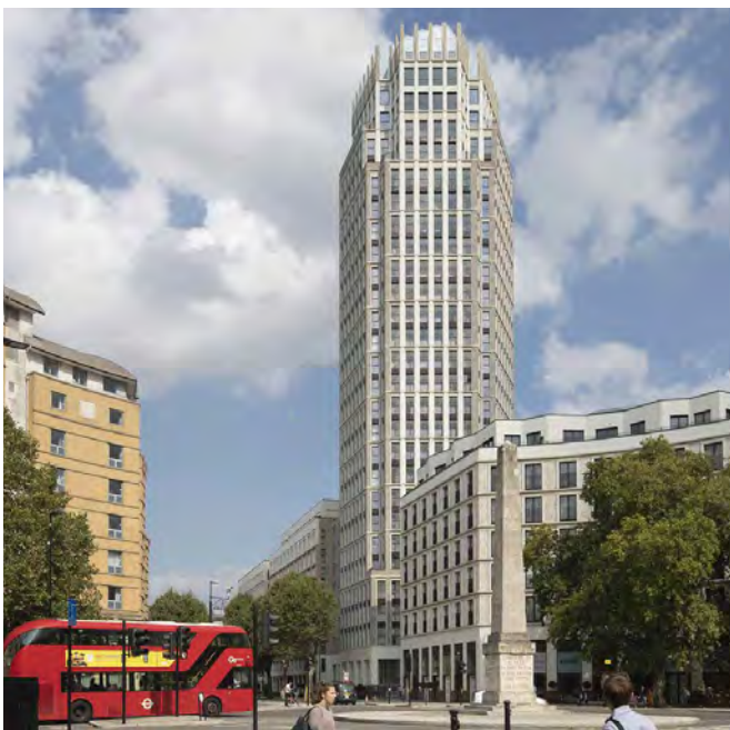
Fig. 299: Blackfriars Circus, 'The use of brick cladding on this tall building gives it a character that fits well into its historic surroundings, and a texture that is human scale and tactile where the building meets the ground.'
