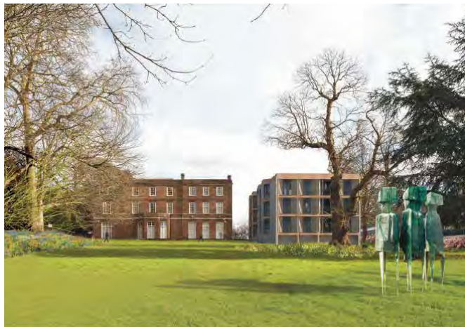
Fig. 357: Chadwick Hall scheme image © Henley Halebrown Rorrison architects (Design & Access Statement, 2013)
