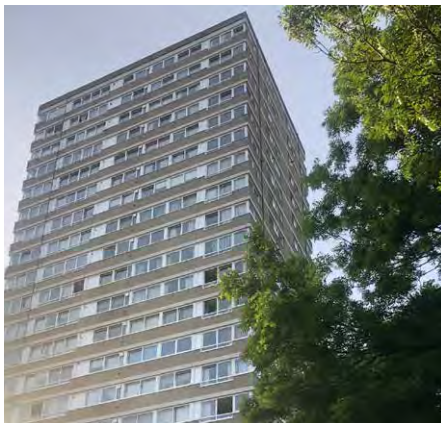
Fig. 83: A 21 storey tower in the Surrey Lane Estate
