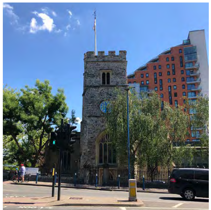
Fig. 302: St Mary's Church next to Putney Bridge is overwhelmed by the adjacent Putney Wharf Tower
