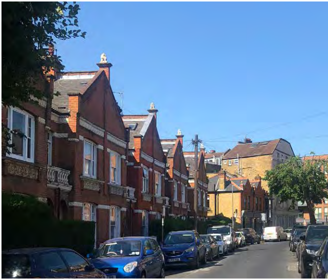
Fig. 73: Consistent red brick terraced houses in Dinsmore Road Conservation Area. Modern infill developments at the end of the road
