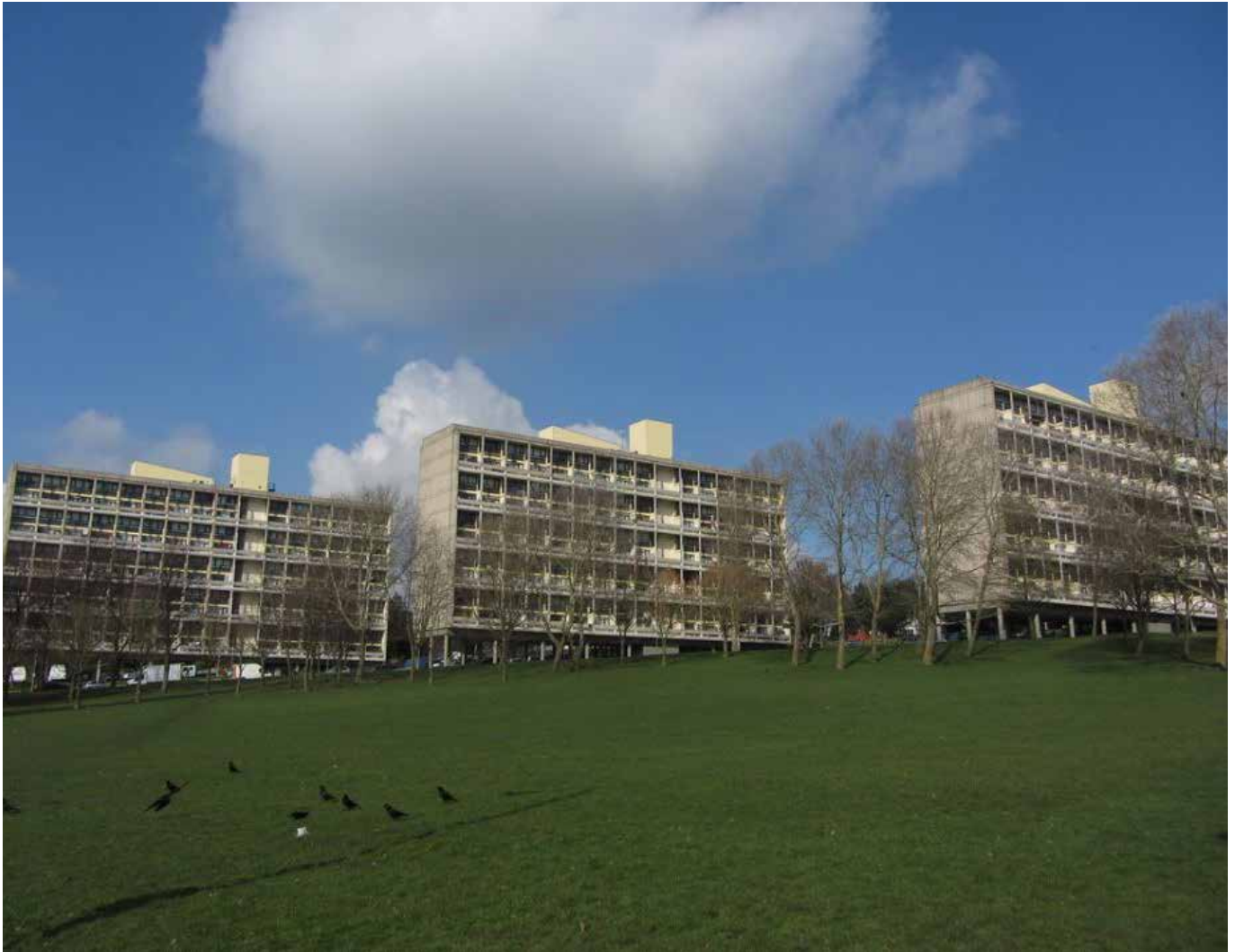
Fig. 175: The listed concrete estates of the post war era are a key characteristic of Roehampton
