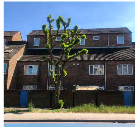
Fig. 85: Low density 3 storey houses to the south of York Road.
