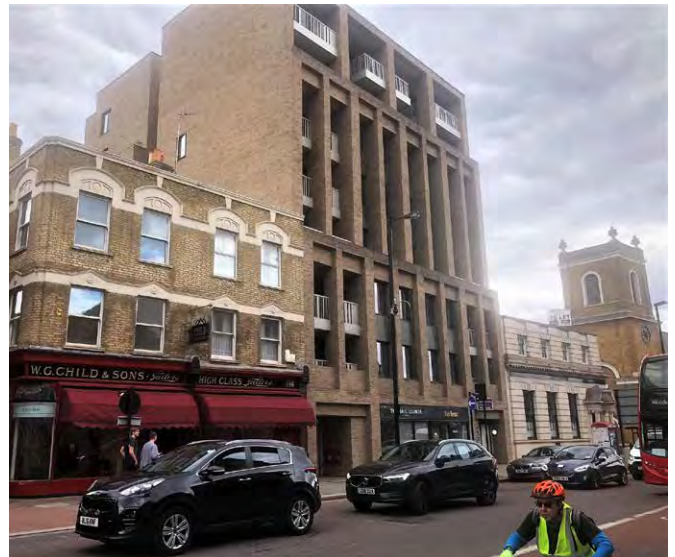
Fig. 342: While the detailing of this building along Wandsworth High Street uses sympathetic materials, its mass conflicts with the proportions of the street and the landmark heritage asset of the church to the right.
