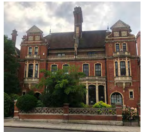
Fig. 77: Landmark villas 69-79 Nightingale Lane (grade II listed)
