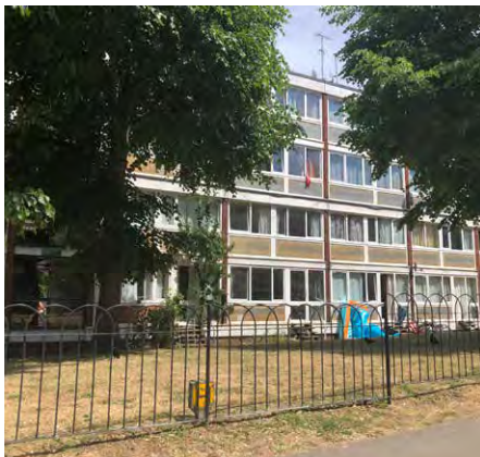
Fig. 185: Bland amenity grass in front of the 4 storey block creates a poor frontage to Danebury Avenue
