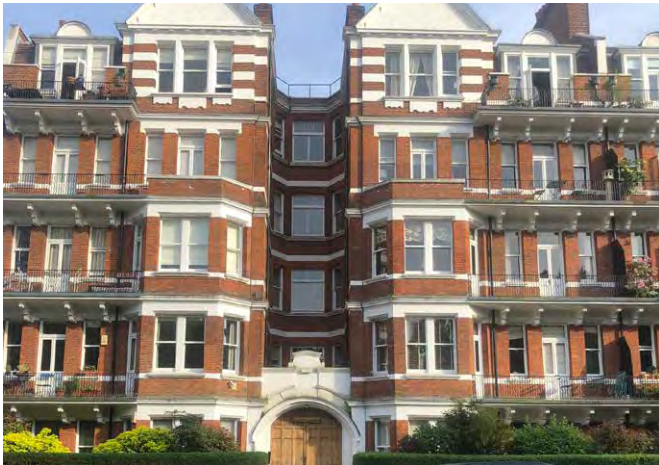
Fig. 380: Mansion blocks fronting Battersea Park
