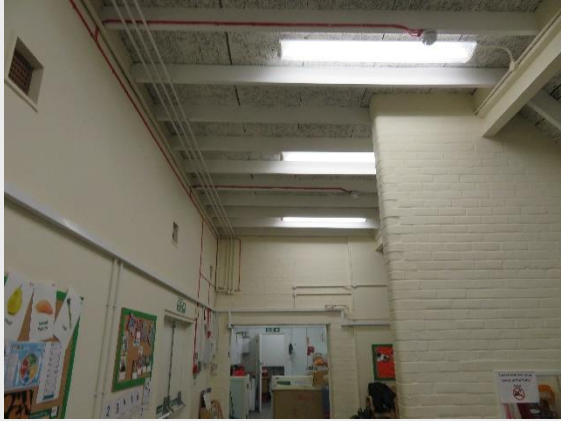
Photograph 1. Underside of roof in the centre
