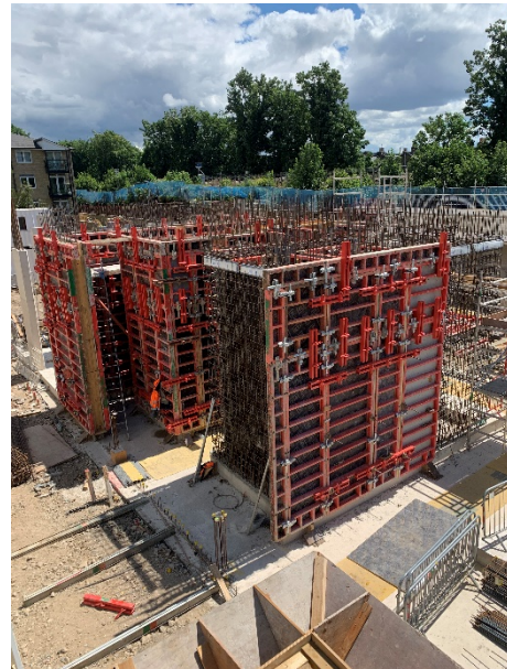
Block D Lift & Stair Core
