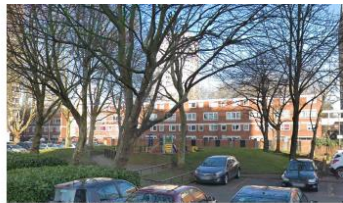
EXISTING CONDITIONS AT FRASER COURT
