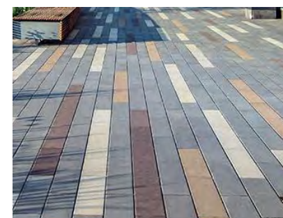
Area A Paving to entrance areas
