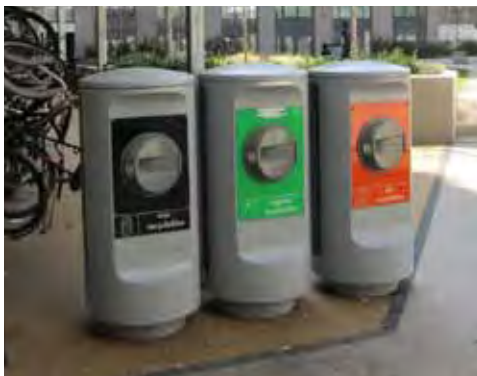
Figure 9.5: pneumatic waste collection system at Wembley
