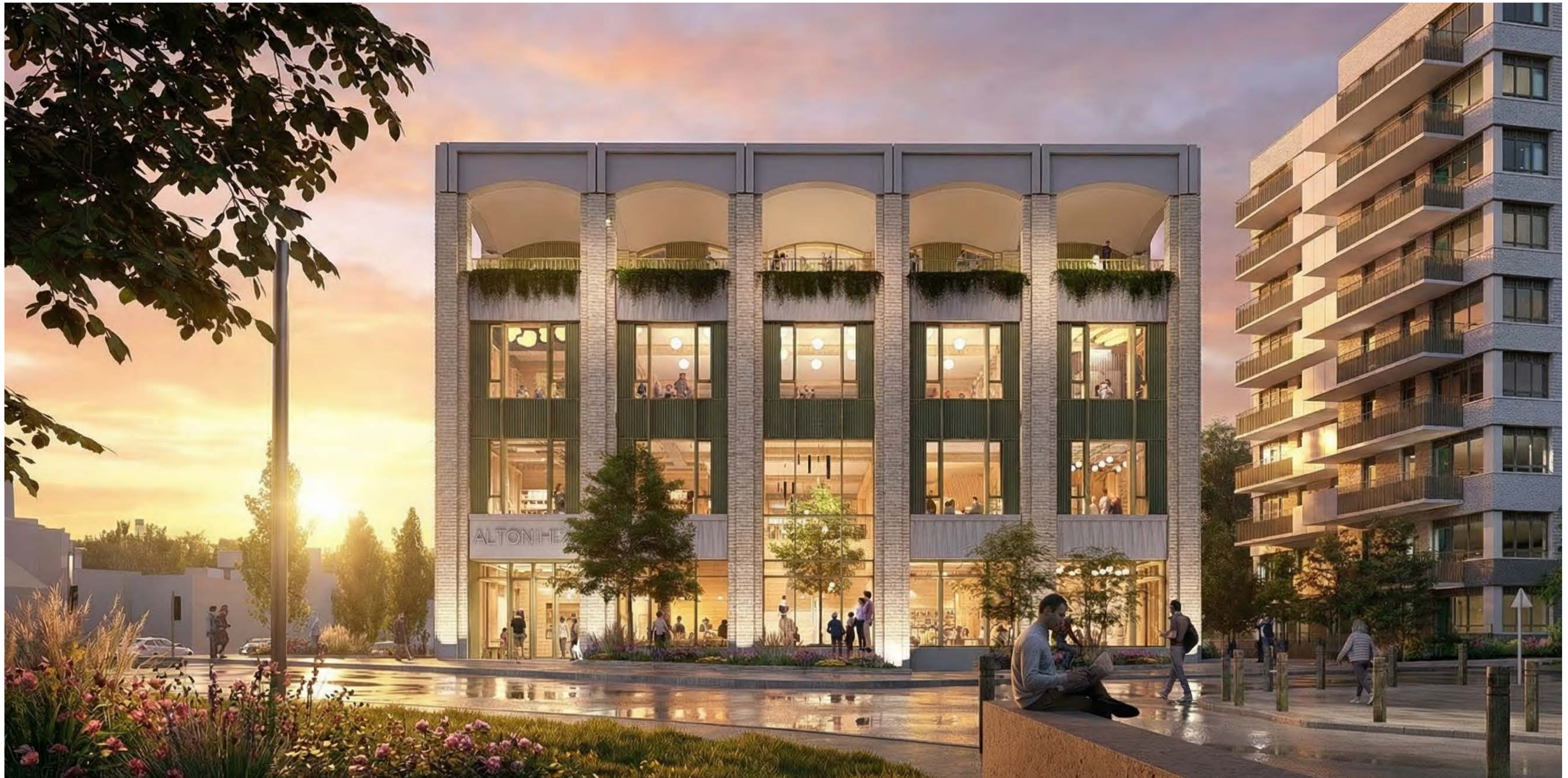
View from Danebury Avenue
