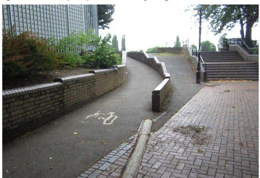
Figure 5.4: The steep ramp with little safety and guidance features
