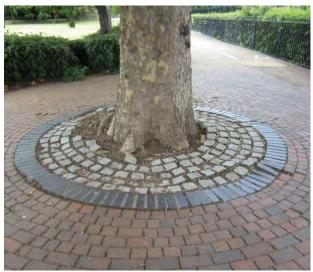
Uneven granite setts and paving due to tree roots.
