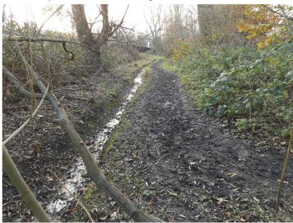
7.15 This channel terminates just before the railway crosses over the cycleway/footpath and the ditch discharges into a small headwall/inlet as shown below. This arrangement looks prone to permitting leaf-litter to be carried into the downstream drain through the inlet opening though the small scale of the feature would make total exclusion of such matter very difficult indeed without risking total blockage and potential flooding of the adjoining path.
