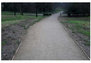
Newly installed compacted hoggin path
