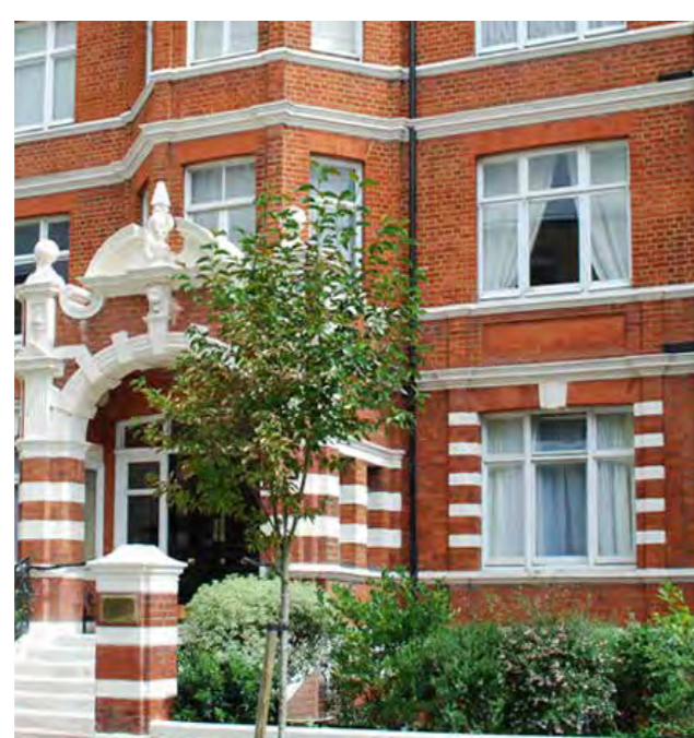
Raised floor provides natural privacy
