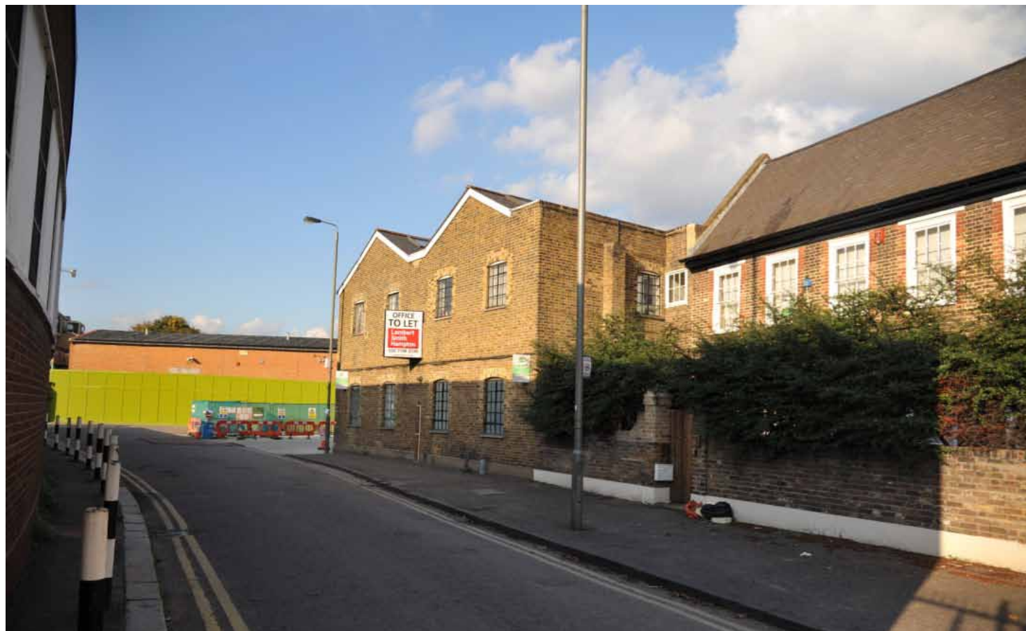
Photo 11 Office Annex to Wentworth House (2 storeys with Conservation Area)
