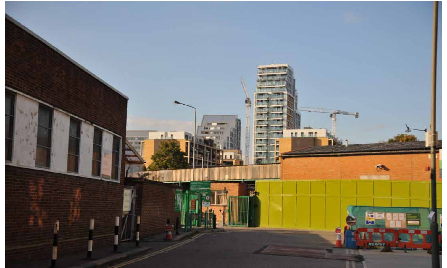
Photo 14 Larger scale massing to North beyond elevated railway line
