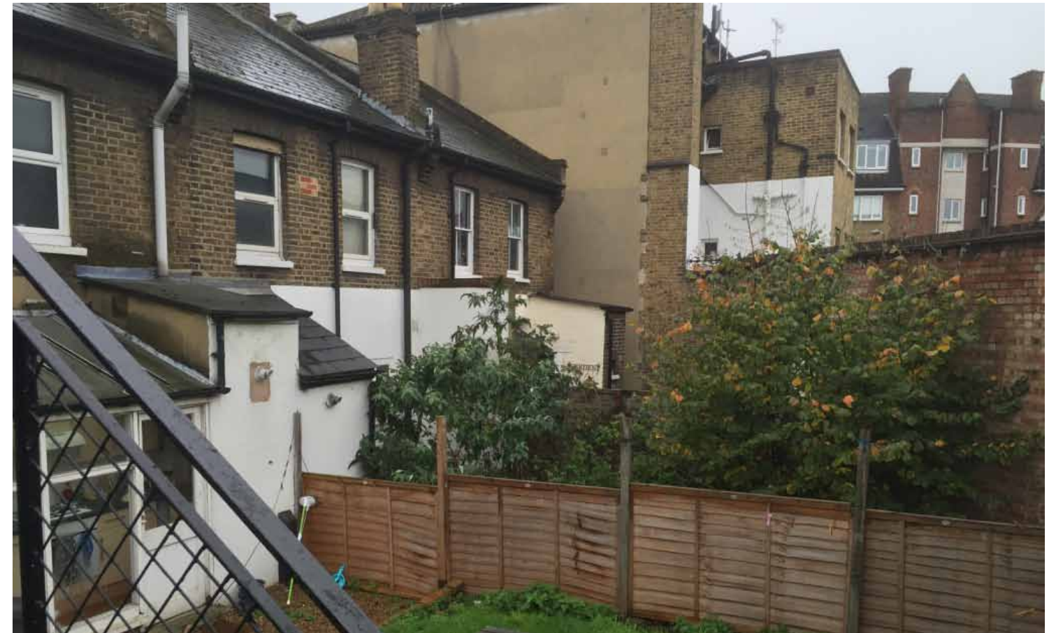
Photo 16 Windows to rear elevations of 16-20 Armoury Way
