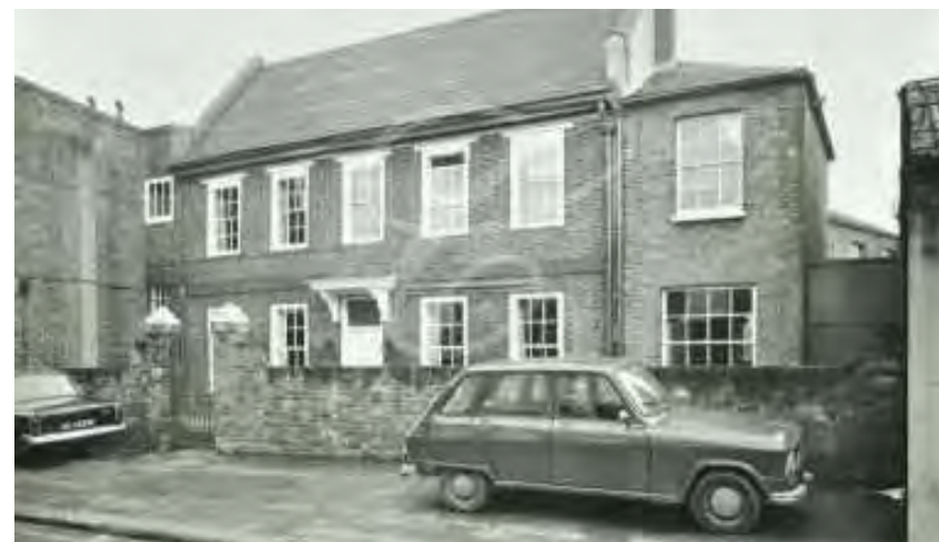
Grade II Wentworth House opposite Panorama Antennas's building
