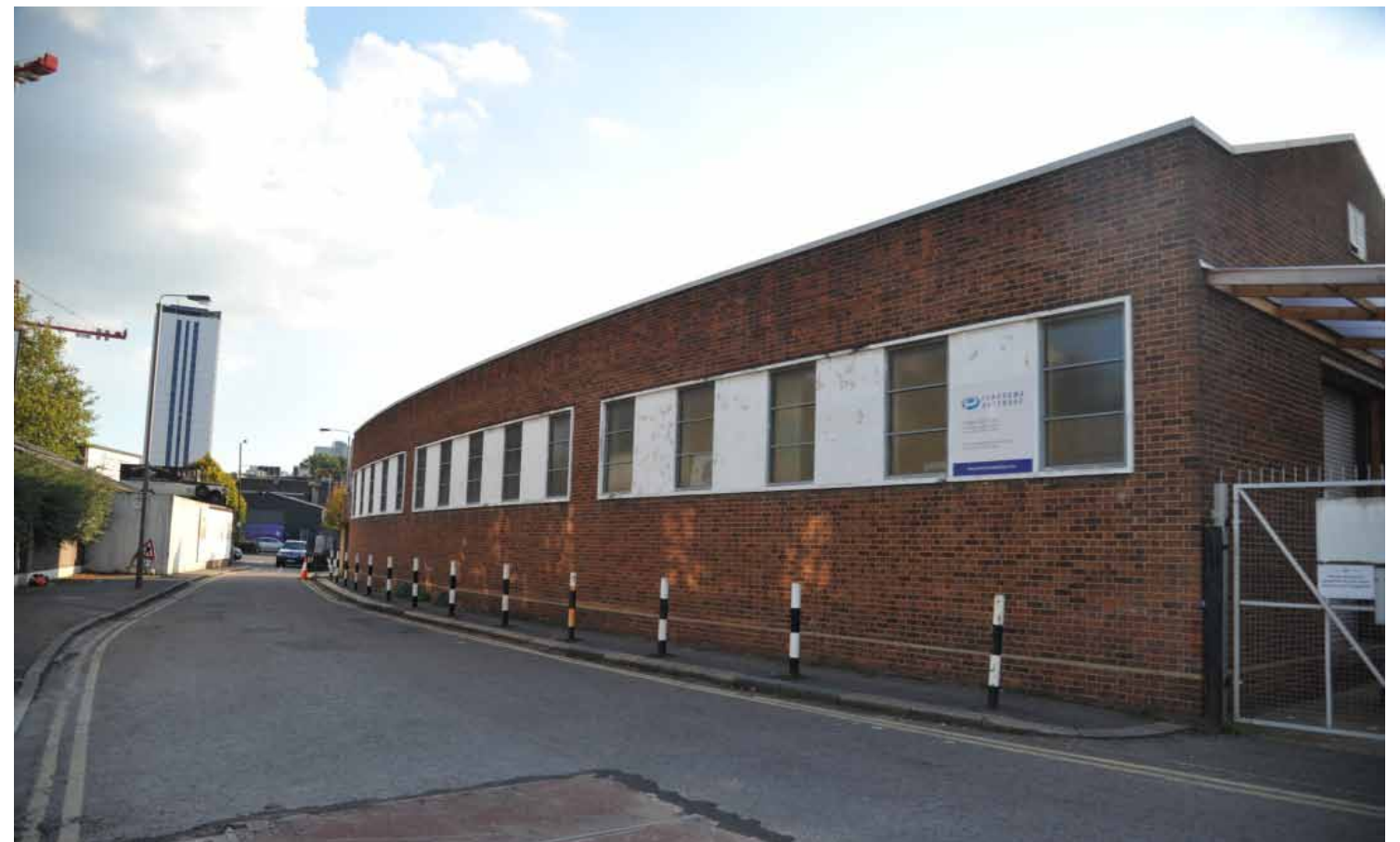
Photo 12 Rear Elevation of Panrorama Antennas Parts storage Warehouse on Dormay St NB Closed/inactive elevation does not contribute to street scene
