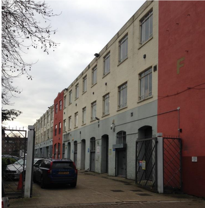
B1 office/studio units for SMEs at Riverside Business Centre
