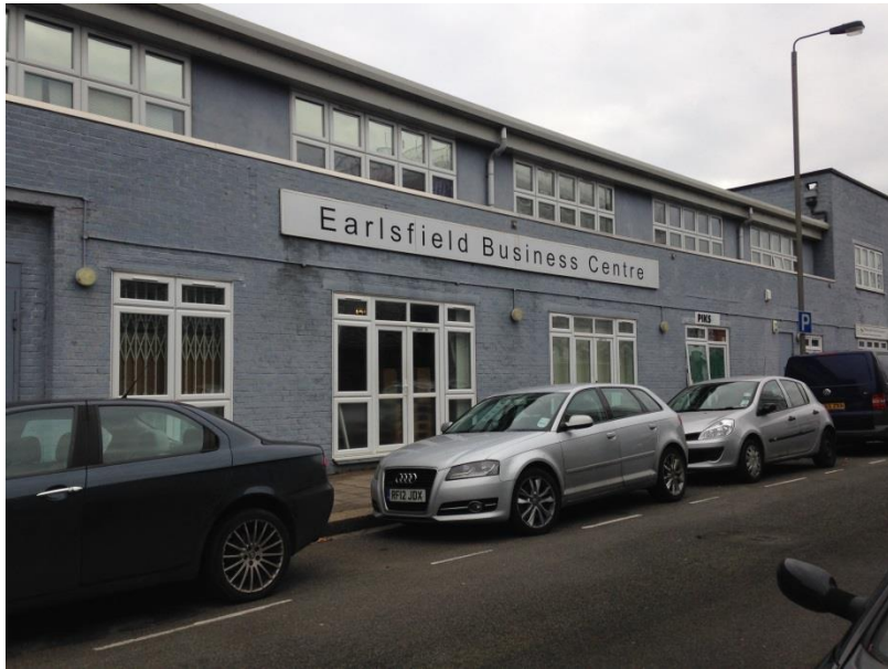
B1 Office units for SMEs at Earlsfield Business Centre
