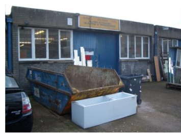
View of buildings from rear
