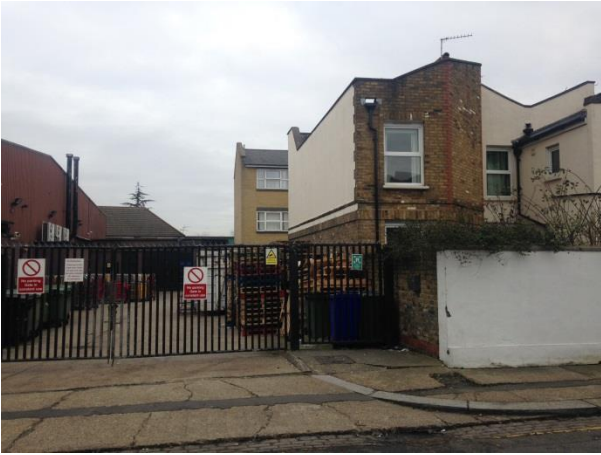
Rear of residential properties within the LSIA
