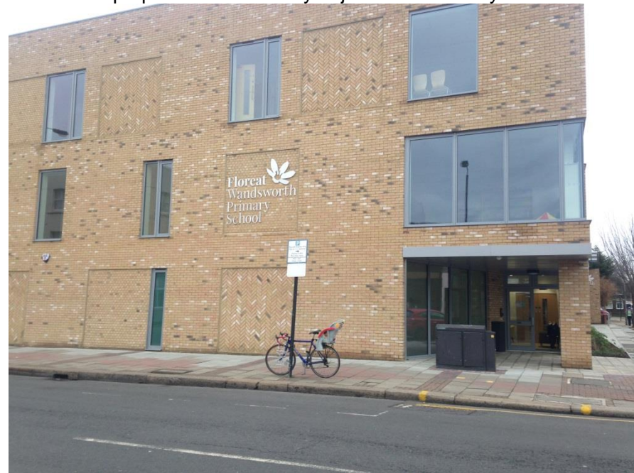
New Floreat Wandsworth Primary School opposite Lydden Road junction
