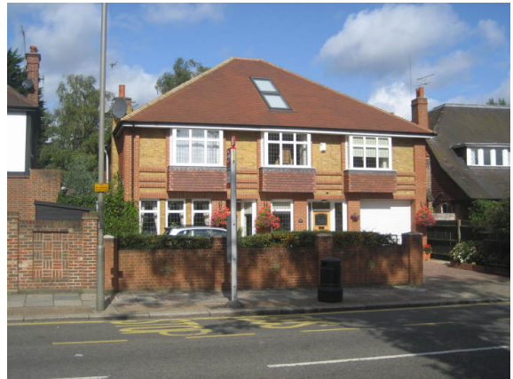
Figure 40 : 400 Wimbledon Park Road
