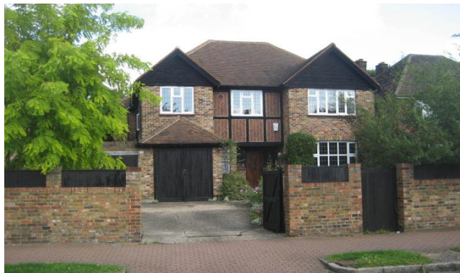
Figure 22 : A house by Alfred Styles showing the characteristic waney edged timber to the gables
