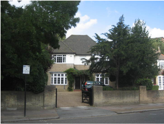
Figure 37 : 386 Wimbledon Park Road
