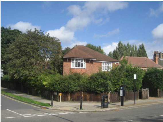
Figure 39 : 394 Wimbledon Park Road
