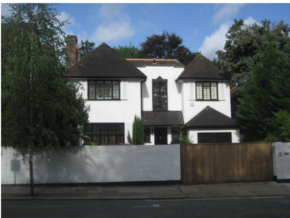
Figure 41 : 404 Wimbledon Park Road
