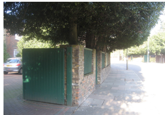
Figure 55 : Timber gate and fence on Inner Park Road
