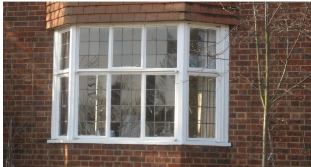
Figure 51 : Bay window with metal frames and small square leaded lights
