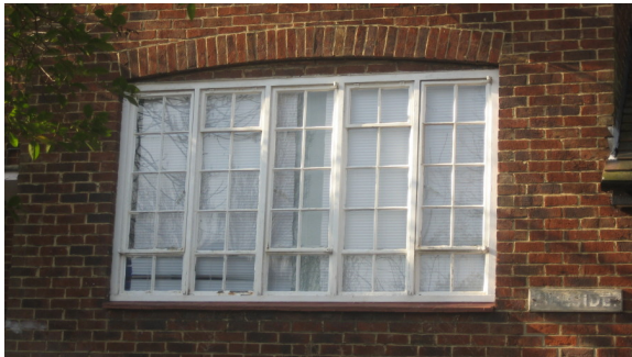
Figure 50 : Crittall windows with steel glazing bars and small square panes
