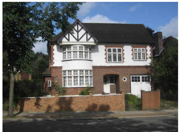
Figure 42 : 406 Wimbledon Park Road
