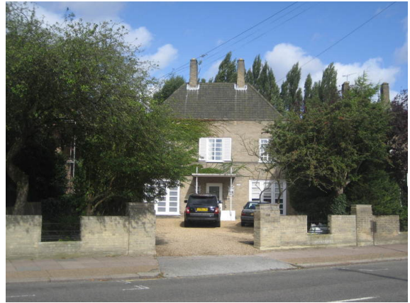
Figure 38 : 390 Wimbledon Park Road
