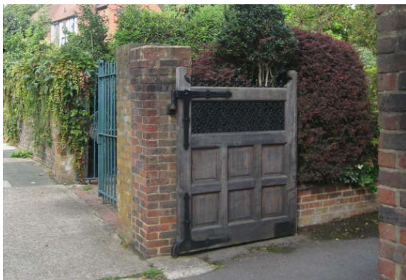
Figure 54 : Timber gate on Woodspring Road
