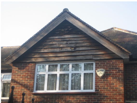
Figure 48 : Waney edge boarding
