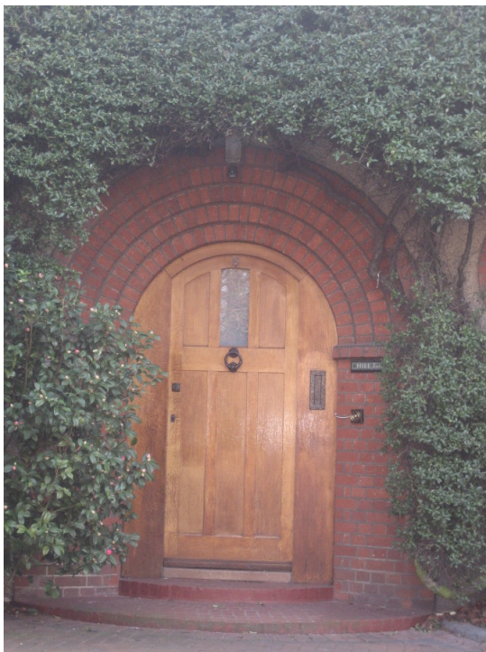
Figure 52 : Oak front door with arch brick surround
