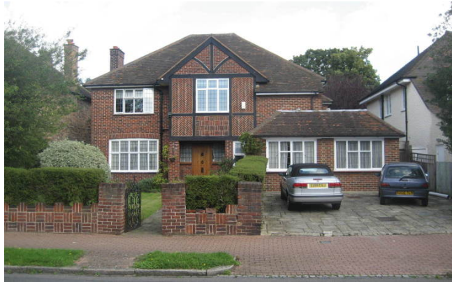
Figure 21 : 6 Kingsmere Road with mock half timbering
