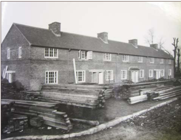
During construction - Laneway
