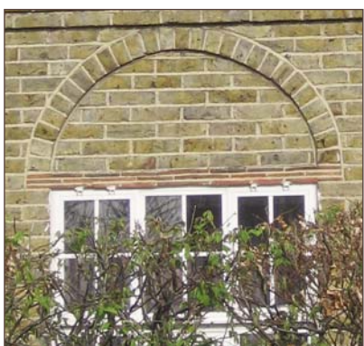
Tile creasing above the windows.
