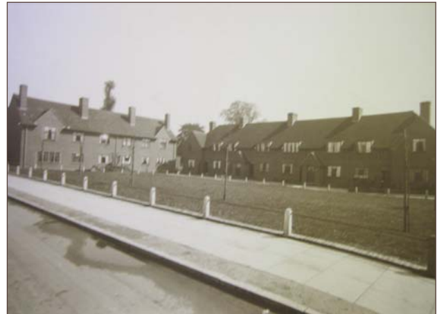
Dover House Road - soon after construction
