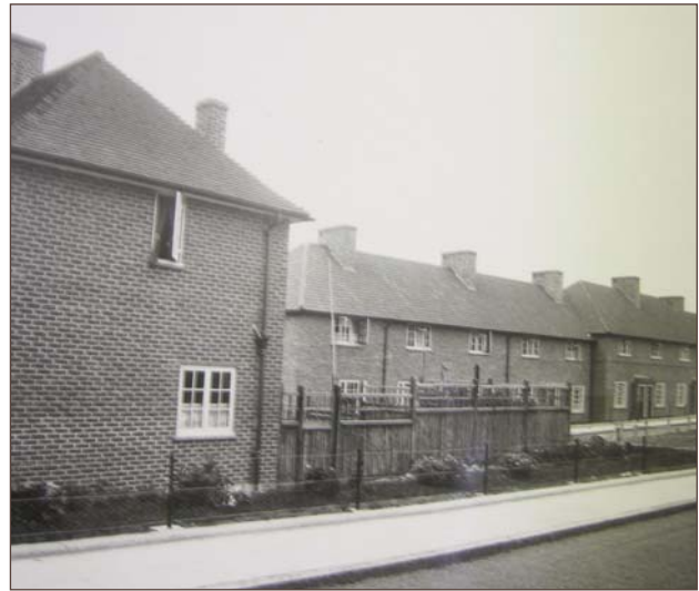
An original boundary fence with trellis to a rear garden. Note: strained wire fence protecting the new hedge.
