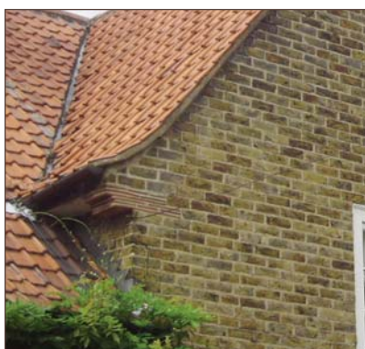
Tile creasing by the eaves.
