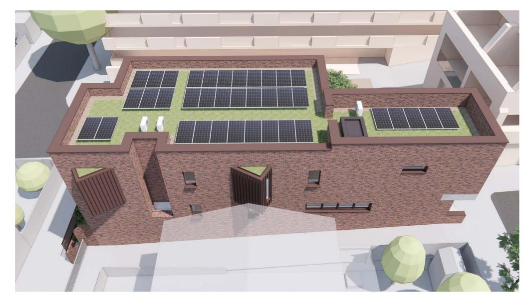
Projecting windows offer directional views and passive surveillance of the rear pathway. Skylights bring light into the building while minimising overlooking
