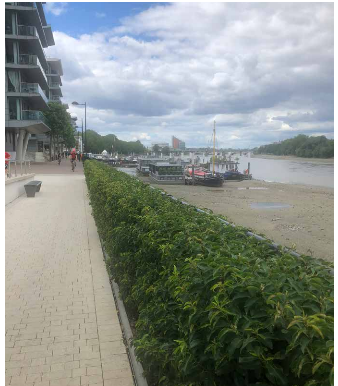
Fig. 304: Along Wandsworth's riverside the design and width of the Thames Path feels like a private space for residents rather than an important continuous public resource for London
