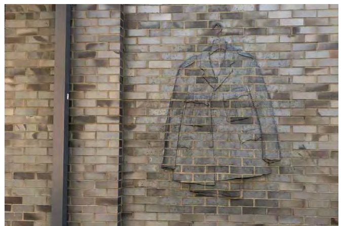
Fig. 300: Careful use of brick detailing within the semi-public space at the base of this development (Peabody Estate, St John's Hill) near Clapham Junction provides a human scale to the building.
