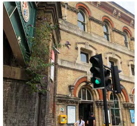
Fig. 97: Grade II listed Battersea Park Station (1865), of pale gaults with detailed stone and red brick details; and the grade II listed railway bridge
