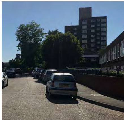
Fig. 180: Low-rise and high-rise estates at Arabella Drive
