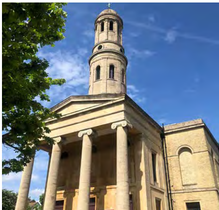
Fig. 225: Landmark Grade II* listed St Ann's Church
