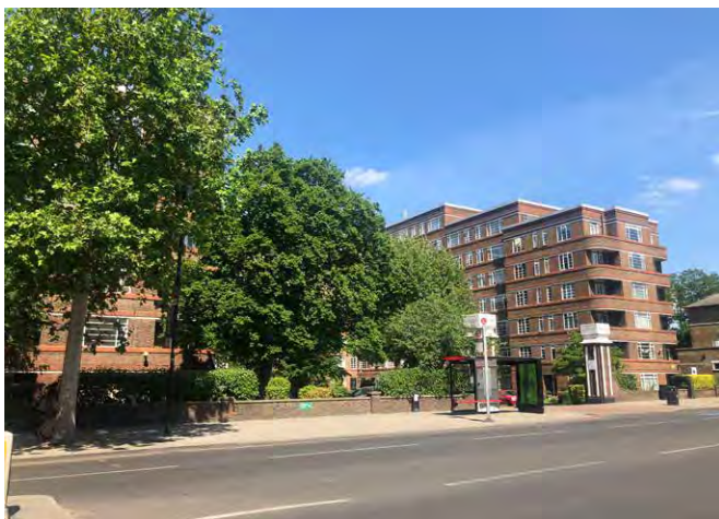
Fig. 296: Du Cane Court in Balham, at eight storeys is taller than the prevailing building heights in the area of 3-4 storeys, but it successfully integrates through stepping down and being well integrated with trees and planting. It is well-sited on the wide Balham High Road.
