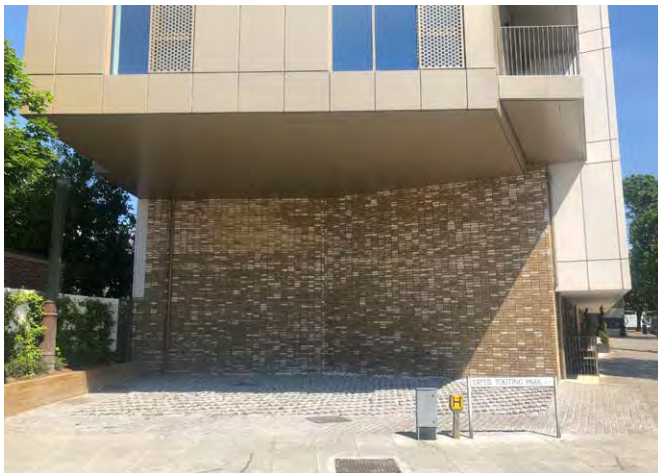
Fig. 307: An example of a poor ground floor frontage at a development on the corner of Balham High Road and Upper Tooting Park
