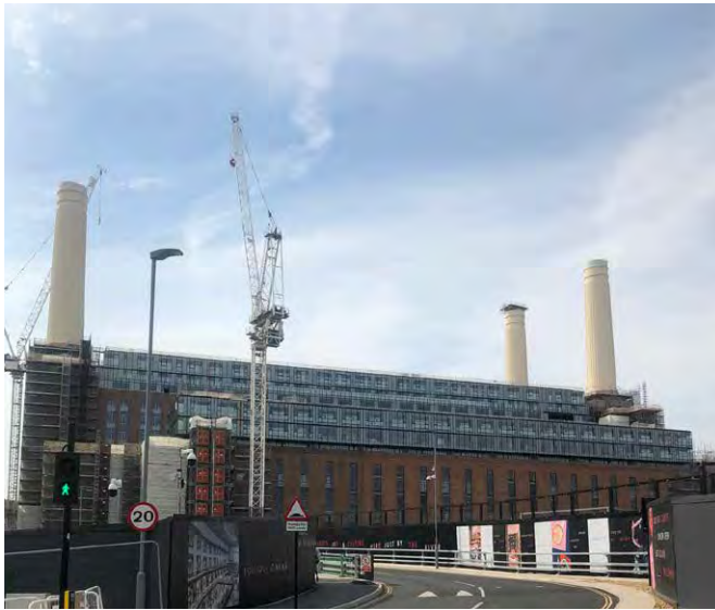
Fig. 93: The iconic Battersea Power Station during redevelopment
