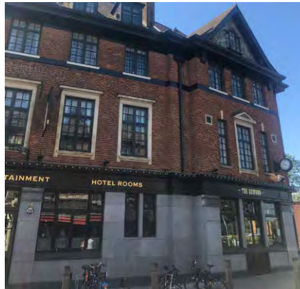
Fig. 70: The Bedford pub is a strong landmark on the corner of Bedford Hill/Balham Station Road
