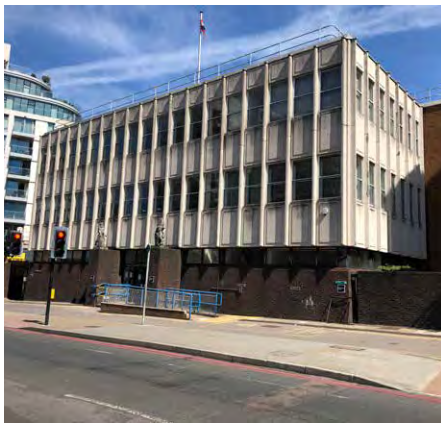
Fig. 141: Commercial buildings with large floor plates along Upper Richmond Road
