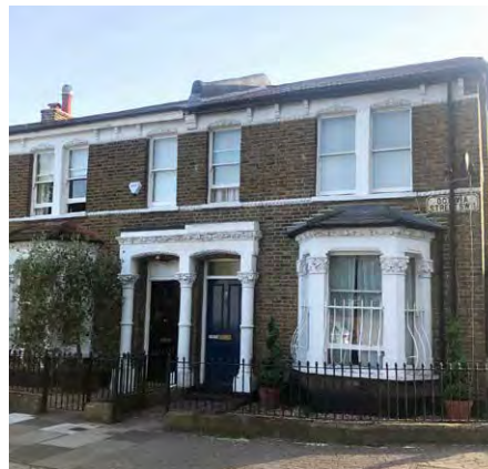
Fig. 84: A traditional mid-Victorian terrace on Octavia St in Three Sisters Conservation Area
