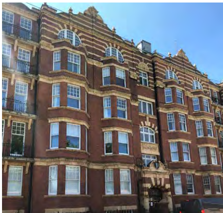
Fig. 147: Kenilworth Court mansion blocks with views across Putney Bridge and the river
