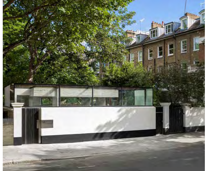
Fig. 339: Earl's court house - A contemporary design on a small site that discreetly slots into a conservation area.
