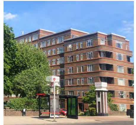
Fig. 71: The Art Deco Du Cane Court forms a strong address to the street. Its gardens provide welcome green to Balham High Road
