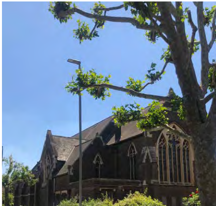
Fig. 211: Locally listed St James Church on Mitcham Lane
