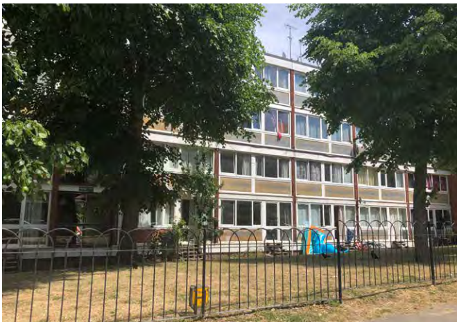
Fig. 381: Mid-rise estate block in Alton East, Roehampton
