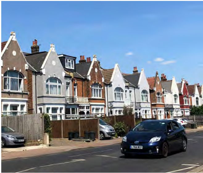
Fig. 209: Two storey terraced houses with cross-gabled roofs on Mitcham Lane
