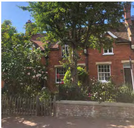
Fig. 171: Cottage style houses on Medfield Street in Roehampton Village Conservation Area
