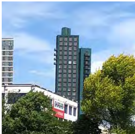
Fig. 353: 11 Mapleton Crescent scheme from King George's Park
