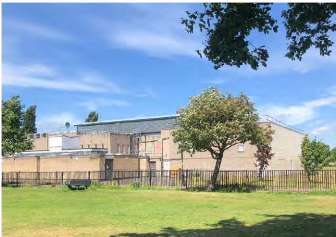
Fig. 390: Large floor plate sub station in Wandle Valley
