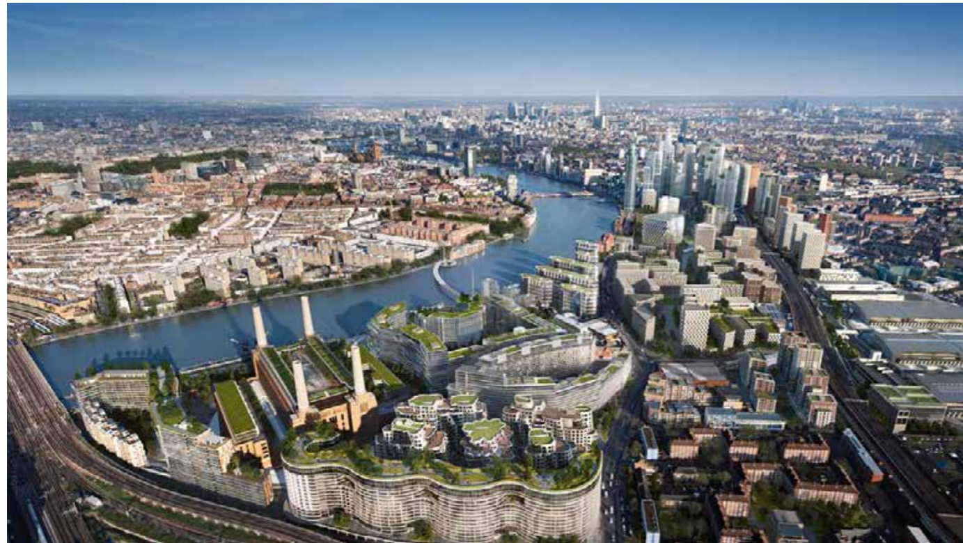
Aerial visualisation showing the preferred location 4C on the Nine Elms Reach of the Thames
