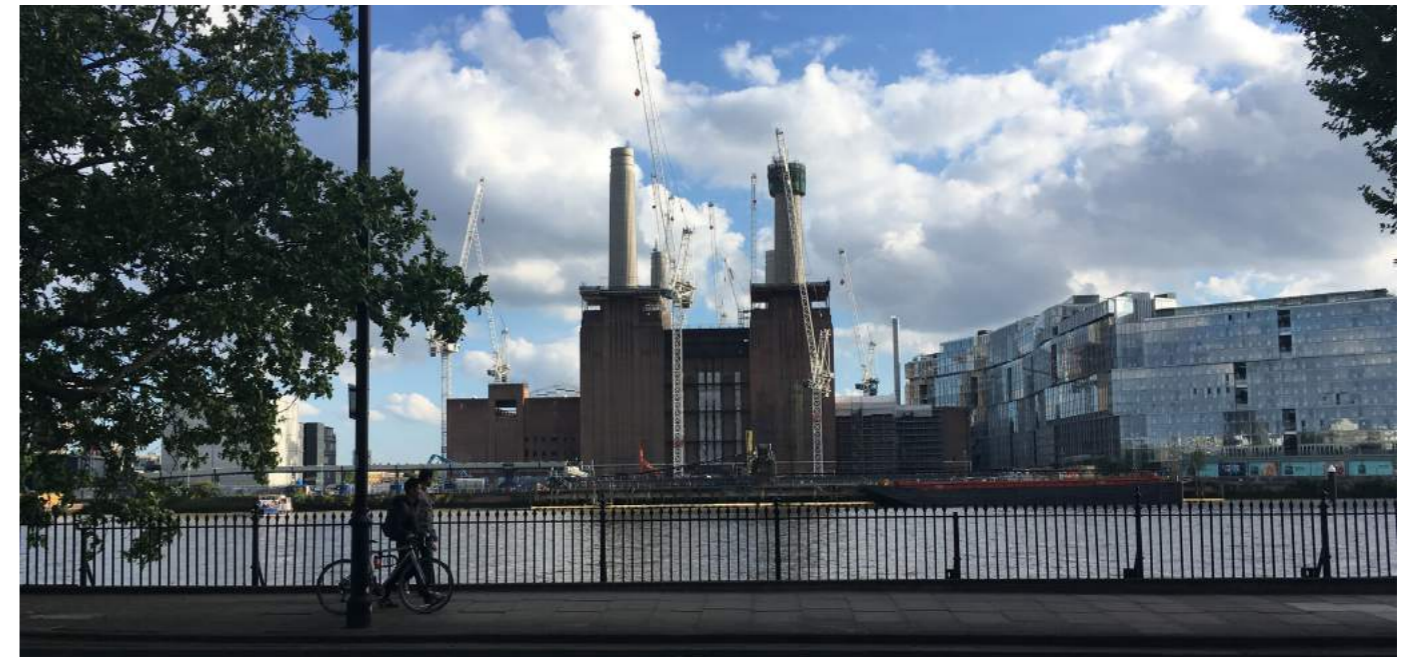
Axial view looking south from the north bank towards the Grade II* Listed Battersea Power Station
