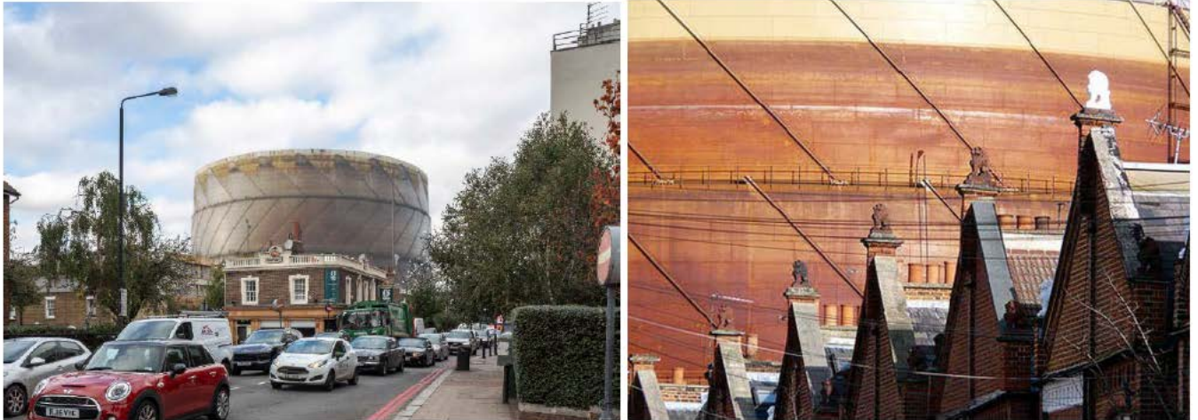
Document 4 - Figure 4-2 The former gasometer, Wandsworth Gasworks
