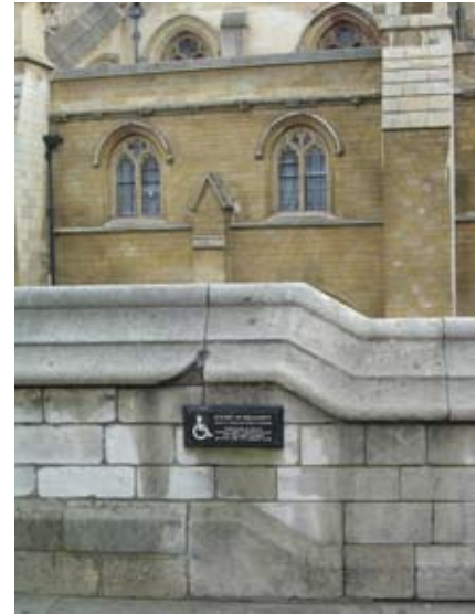
Level access for wheelchair users to the Houses of Parliament involves negotiating a series of complex routes which are signed and at key points attended by staff.
