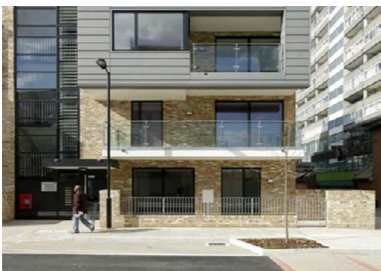
Well lit entrances with no steps and lift access to all homes
