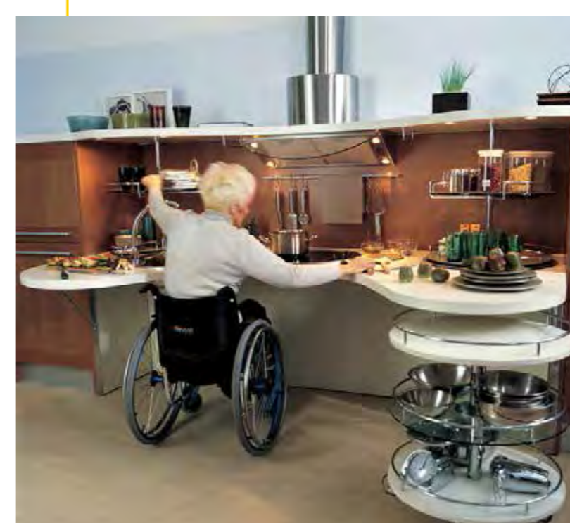
Adjustable height kitchen counter and cupboards in wheelchair flats
