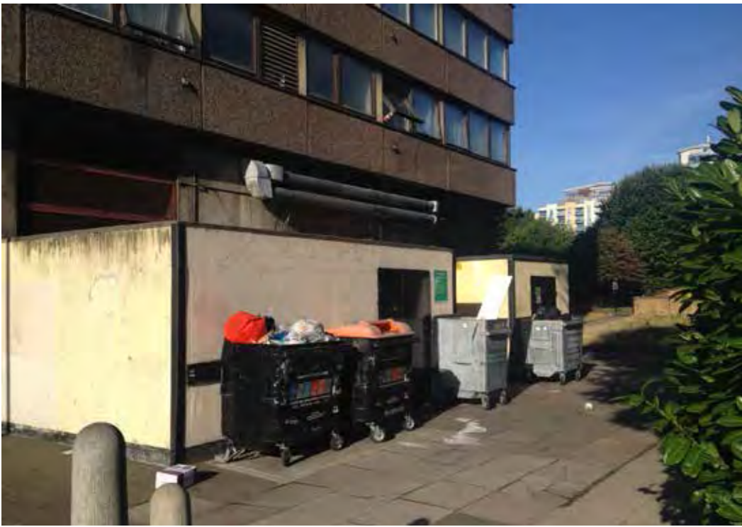
Penge House overflowing refuse store
