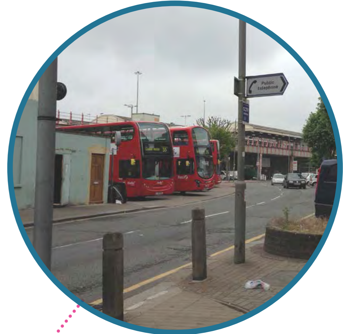
The bus stand creates a barrier and further cuts off the station entrance - visually and physically from Falcon Road
