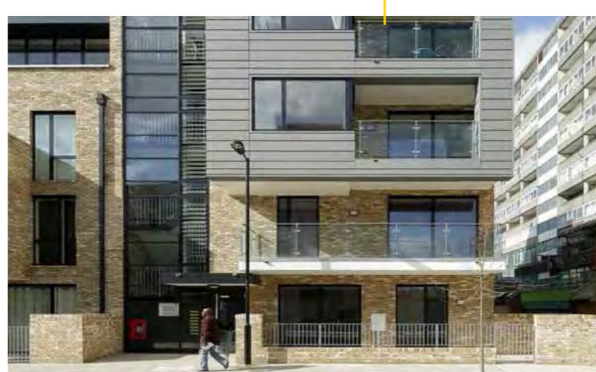
Well lit entrances with no steps and lift access to all homes
