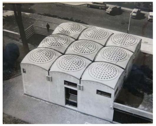
The thin shell concrete roof of Roehampton Library as seen from Allbrook House shortly after completion (LMA)
