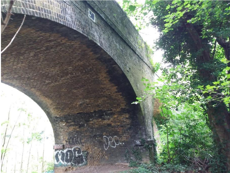
Figure 4.4 Building 1, disused railway viaduct bridge
