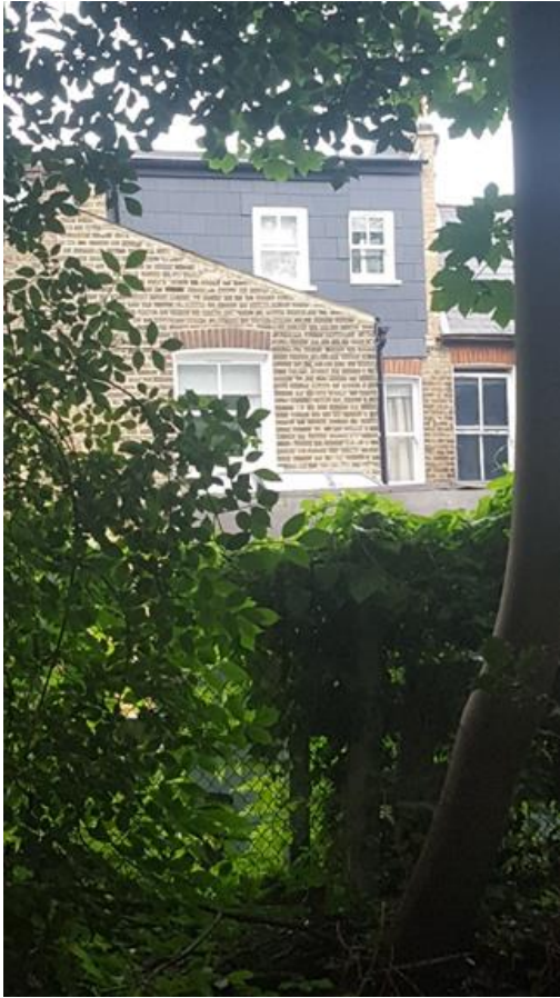
Figure 4.7 Existing south façade of building 3.
