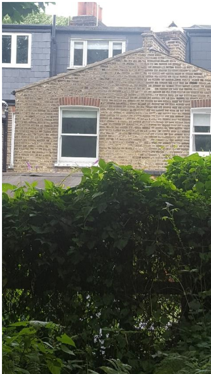
Figure 4.6 Existing south façade of building 2
