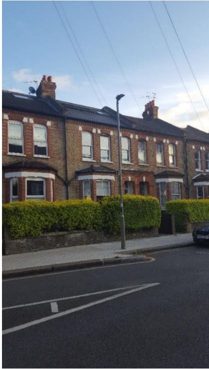
Figure 4.5 Existing north façade of building 2 & 3.
