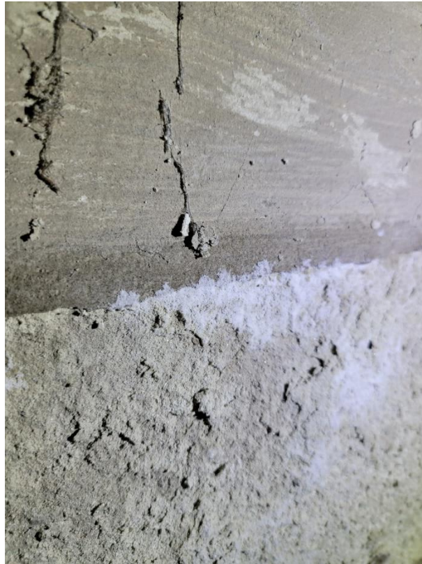
Middle: Photo 17 – Detail of powdering surfaces – Note apparent brush marks in in coating above
