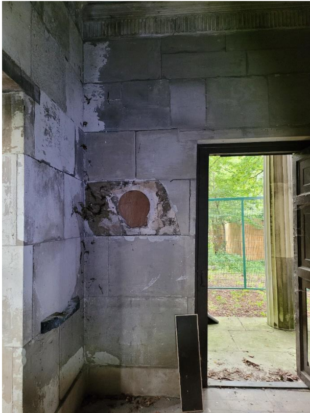
Left: Photo 19 – West elevation – missing/damaged stone behind roundel
