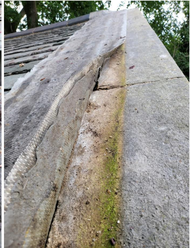
Left: Photo 4 – South roof slope – Westmoreland, diminishing random slating, narrow gutter and felt capping to cornice
