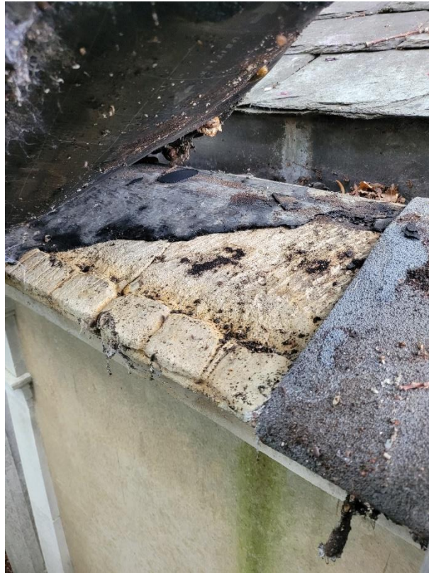
Left: Photo 4 – South roof slope – Westmoreland, diminishing random slating, narrow gutter and felt capping to cornice
