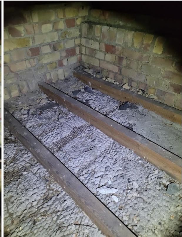
Left: Photo 10 – Roof void – Plaster tray and suspended points added to back of lath and plaster ceiling
