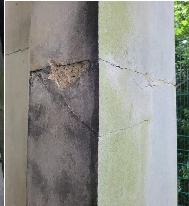
Middle: Photo 2 - North Elevation – note missing downpipe, water runs from gutter and craizing of render
