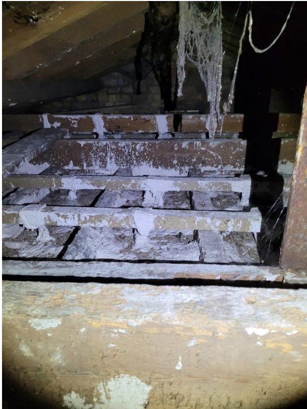
Left: Photo 10 – Roof void – Plaster tray and suspended points added to back of lath and plaster ceiling
