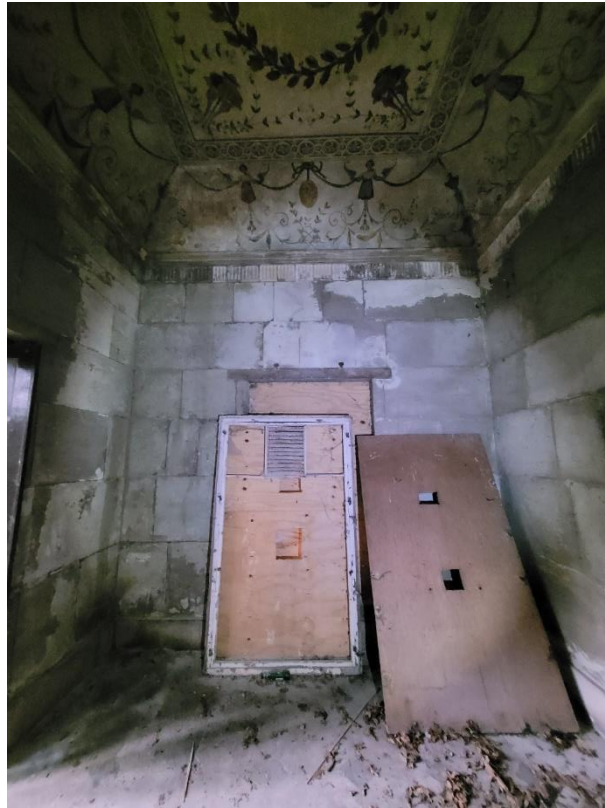
Left: Photo 19 – West elevation – missing/damaged stone behind roundel
