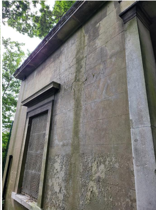
Middle: Photo 2 - North Elevation – note missing downpipe, water runs from gutter and craizing of render
