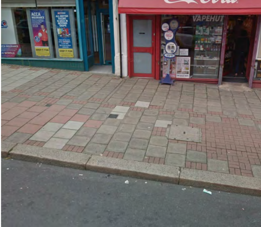
Existing paving in Replingham Road
