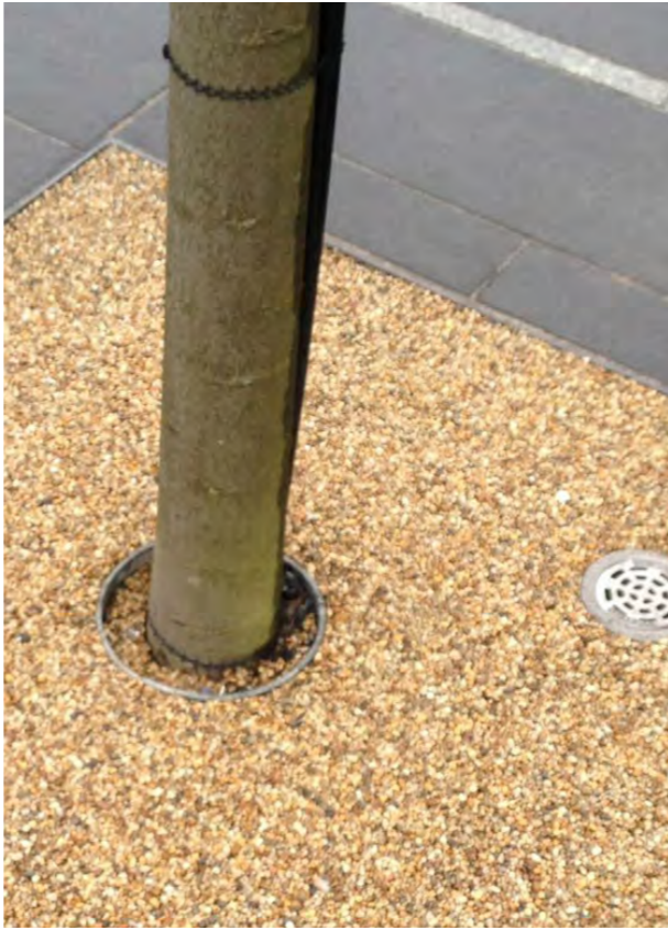
Resin bound gravel at tree pits
