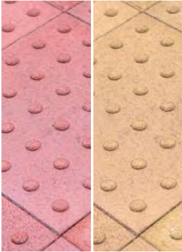
OP.2 Red and buff grey concrete tactile at crossings
