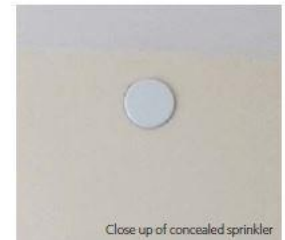
Close up of concealed sprinkler
