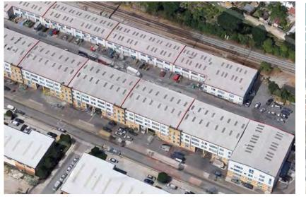
**Stacked Industry (Theydon Road, Hackney)** Smaller industrial units are stacked above larger units through the provision of a ramp serving multiple units at first floor level.
