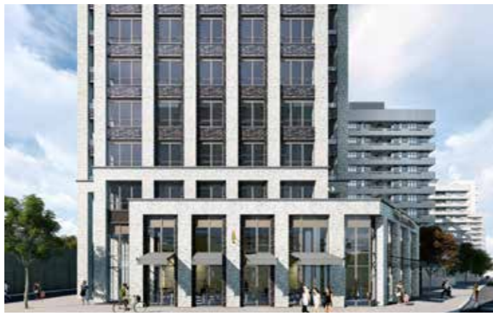
Winstanley Road elevation, Block C
