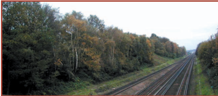
▲ View of train lines from Clapham Junction
