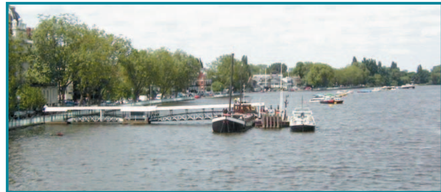
▲ View 1 of Putney Embankment from Putney Bridge
