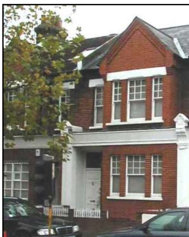
Retained shopfront corbels and fascia framing new ground floor window which mirrors the first floor window above.
