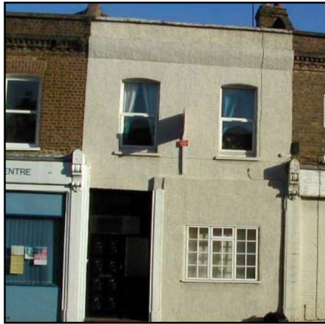
Shopfront fascia removed, small window with horizontal emphasis inserted
