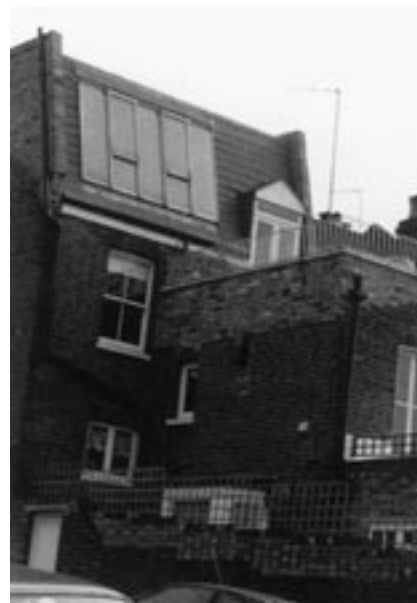
Radical changes to roof shapes, flat roofed extensions and terraces over- looking neighbours are not acceptable
