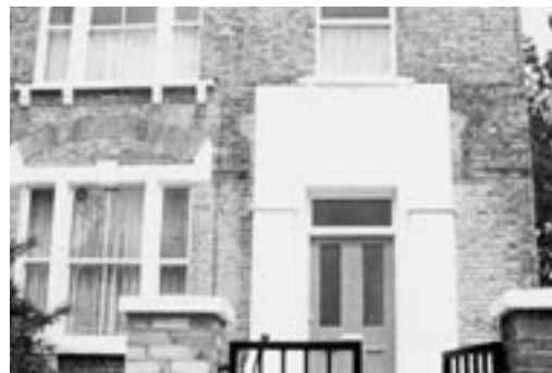
By contrast, a lovely doorcase was removed, and the scar rendered over, where there was no control over it. (Putney)
