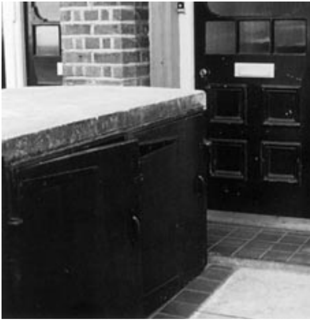
Bin stores should be unobtrusive or even dispensed with – and certainly not block entrances
