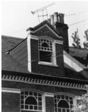
An original dormer – good examples reflect the style and proportions of the house
