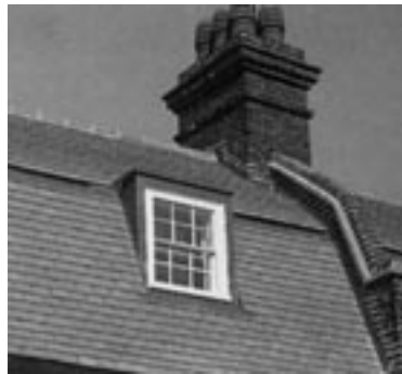
Detail of a new clay tiled roof
