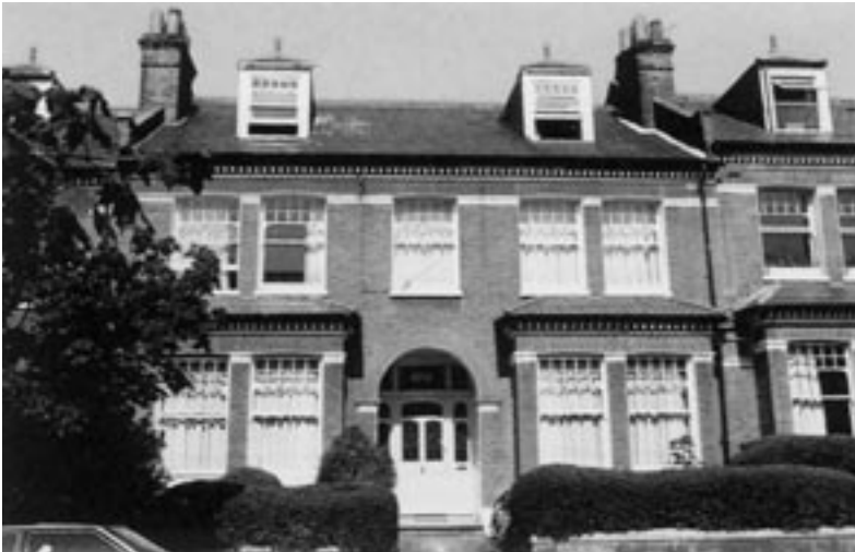
This house retains all the character of its age. (Tooting)
