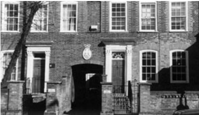
The entire ground floor front of this listed building on the right, has been reinstated following removal of a modern cafe shopfront (Wandsworth)
