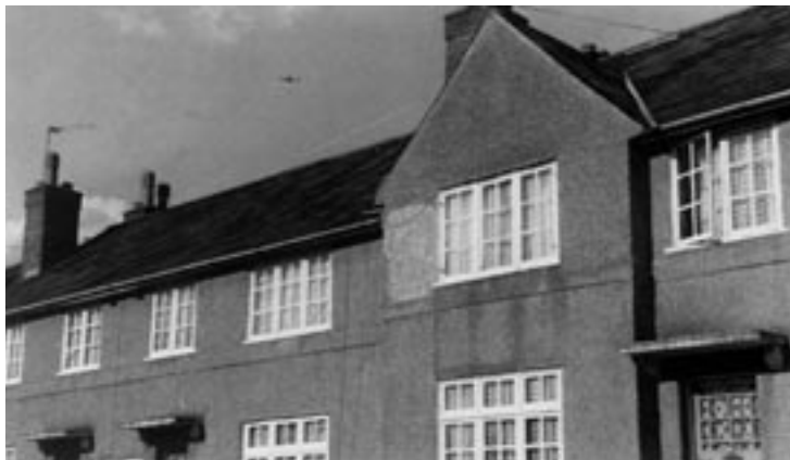
An unaltered group of cottage style houses, finished in unpainted roughcast, but with a poorly matched repair
