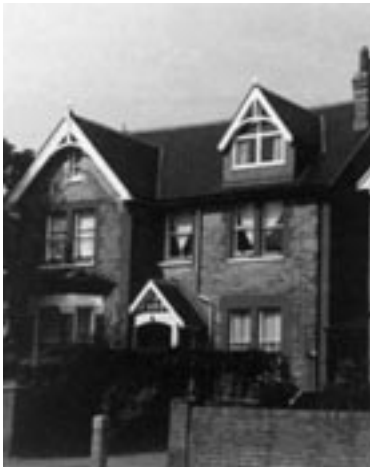
A new dormer – well matched to the original gable (Balham)
