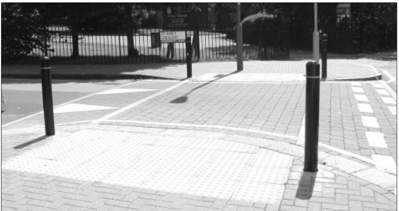
Tactile paving at a raised crossing point, St Ann's Crescent, Wandsworth.
