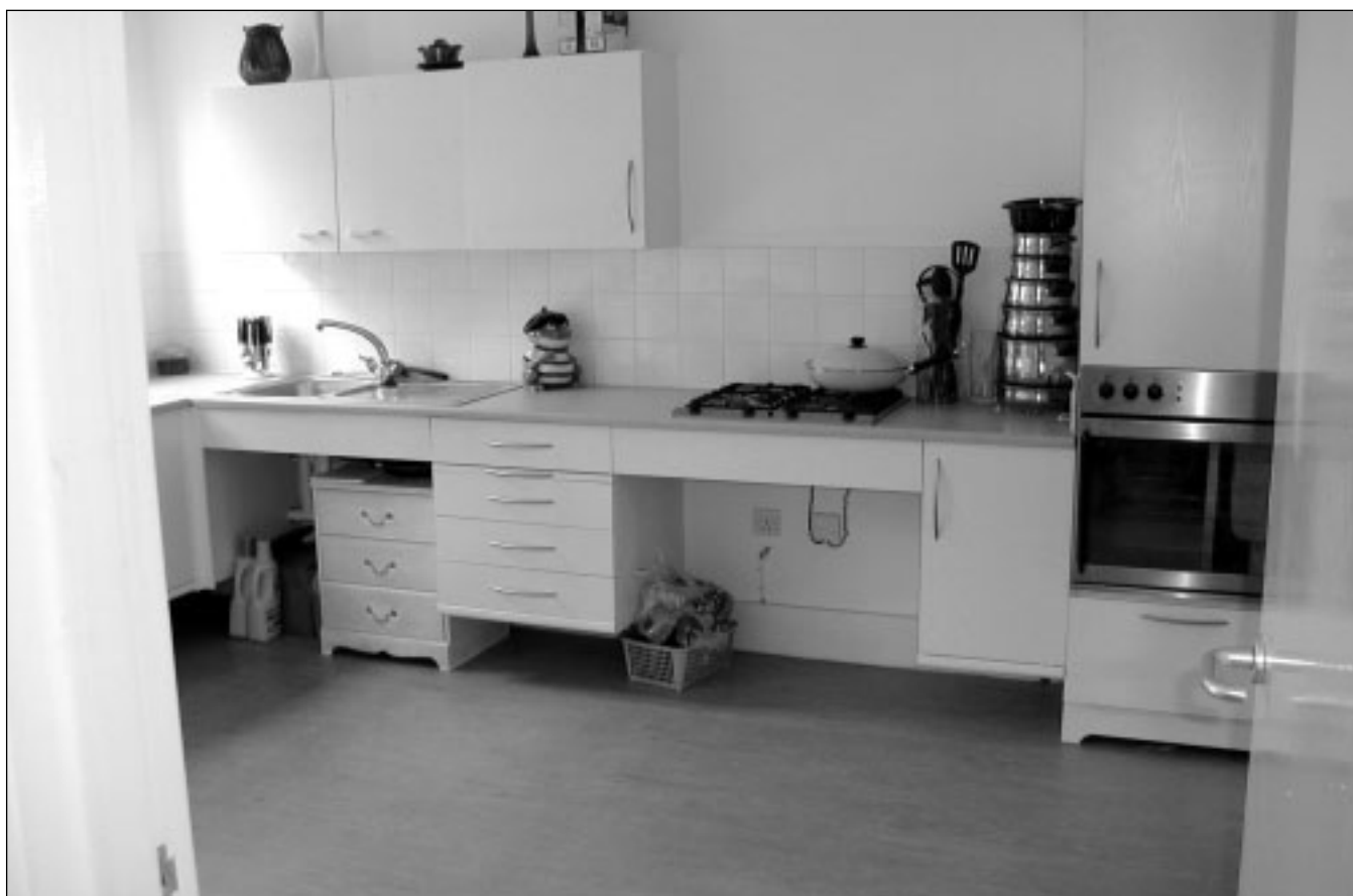
Low level kitchen units and appliances in a housing development.
