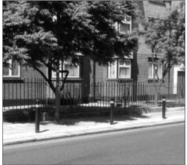
Easily visible Bollard with a colour contrasting collar, Wandsworth Plain
