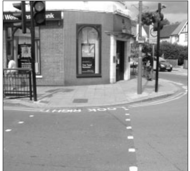
Tactile paving at a dropped kerb at a signal controlled crossing, Wimbledon Park Road, Southfields
