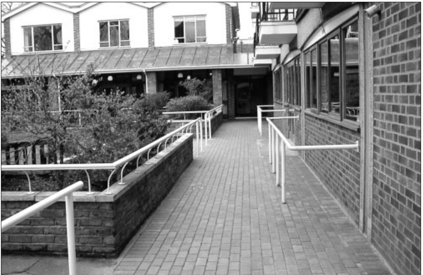
Clearly defined path and guard rails for outward opening windows, Pocklington Court, Roehampton.
