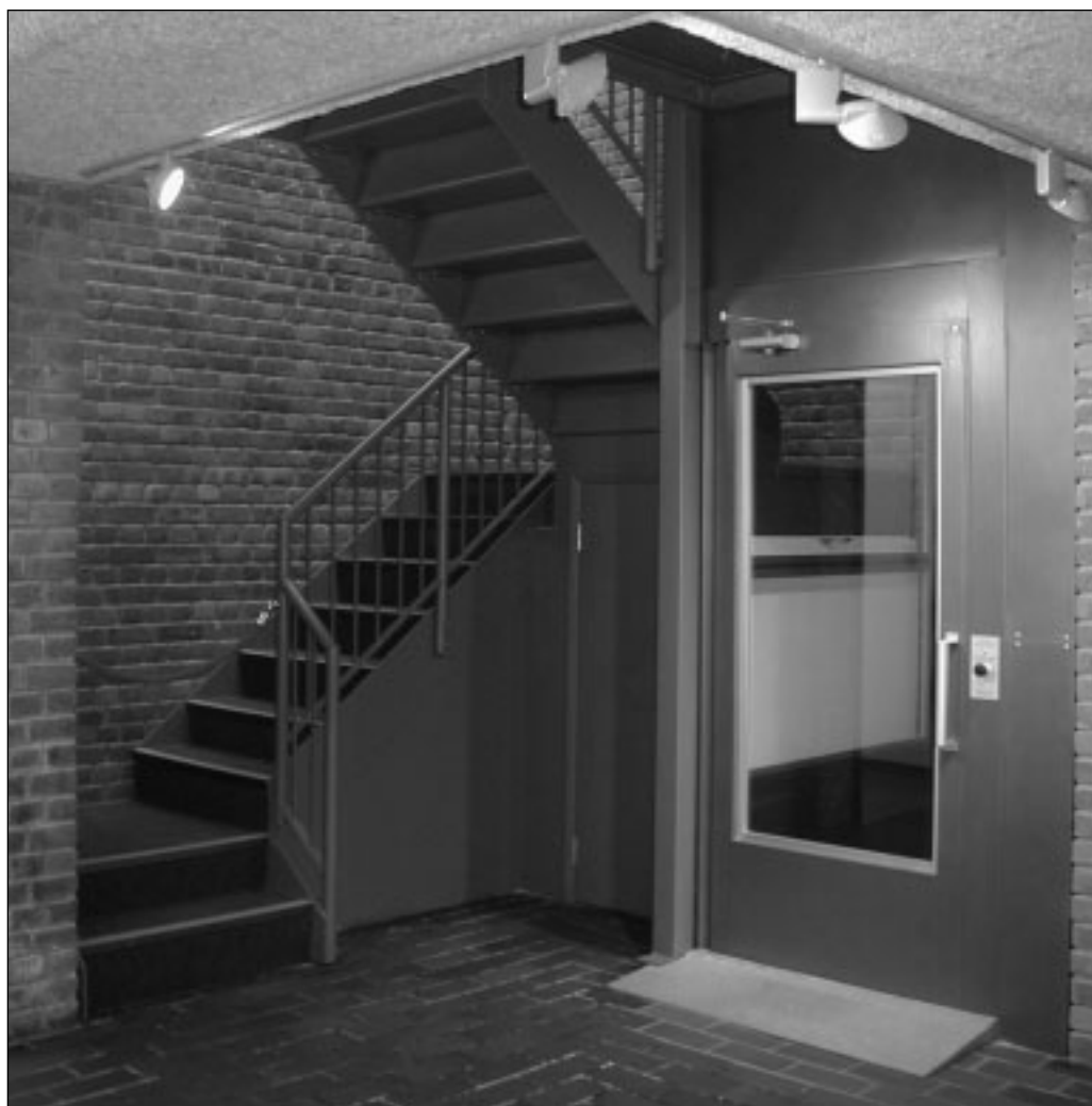
Lift, Battersea Park Library, Battersea Park Road.
