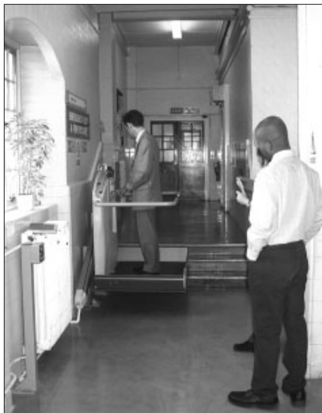
Platform Lift, South Thames College, Wandsworth.
