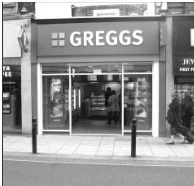
Accessible shopfronts, Greggs, Putney High Street.
