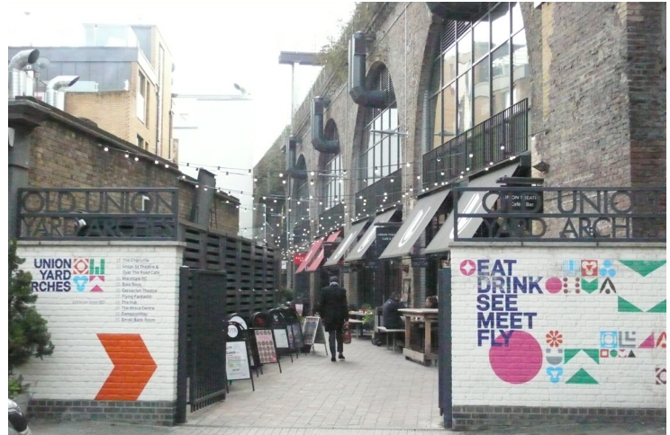
Railway arches and public space
