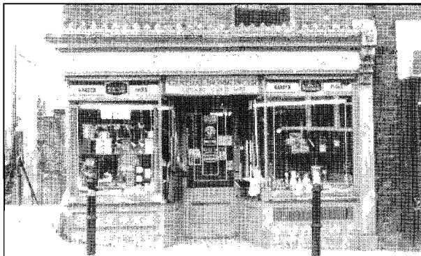
Decorative ironwork applied to cornice
