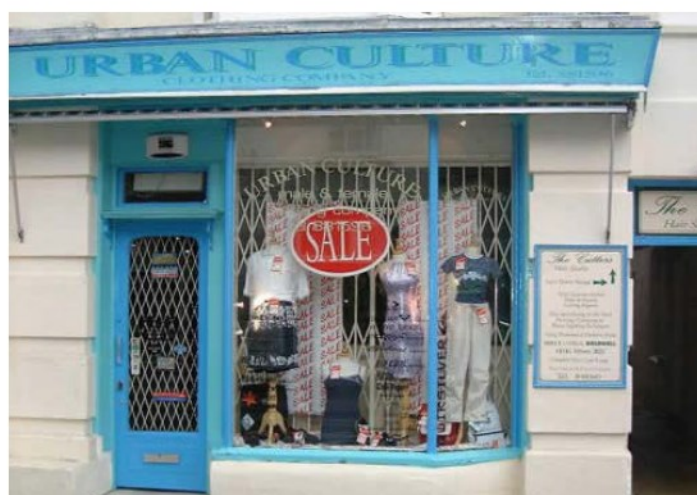
Unobtrusive grilles can provide security while allowing views into shops
