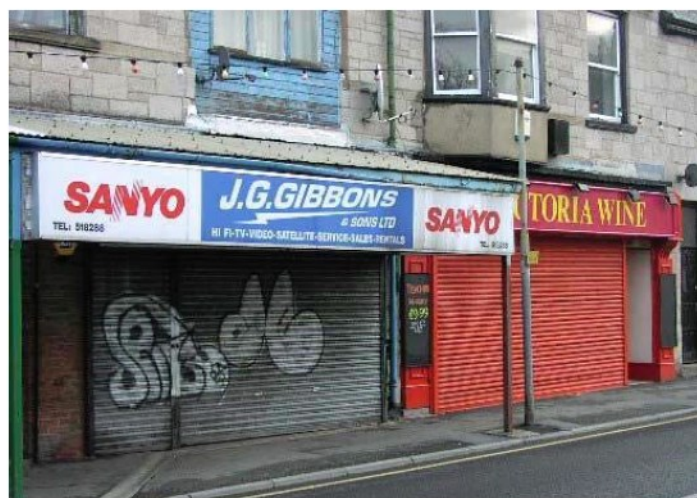
Solid metal shutters can have a detrimental effect on amenity and do not necessarily lead to better security
